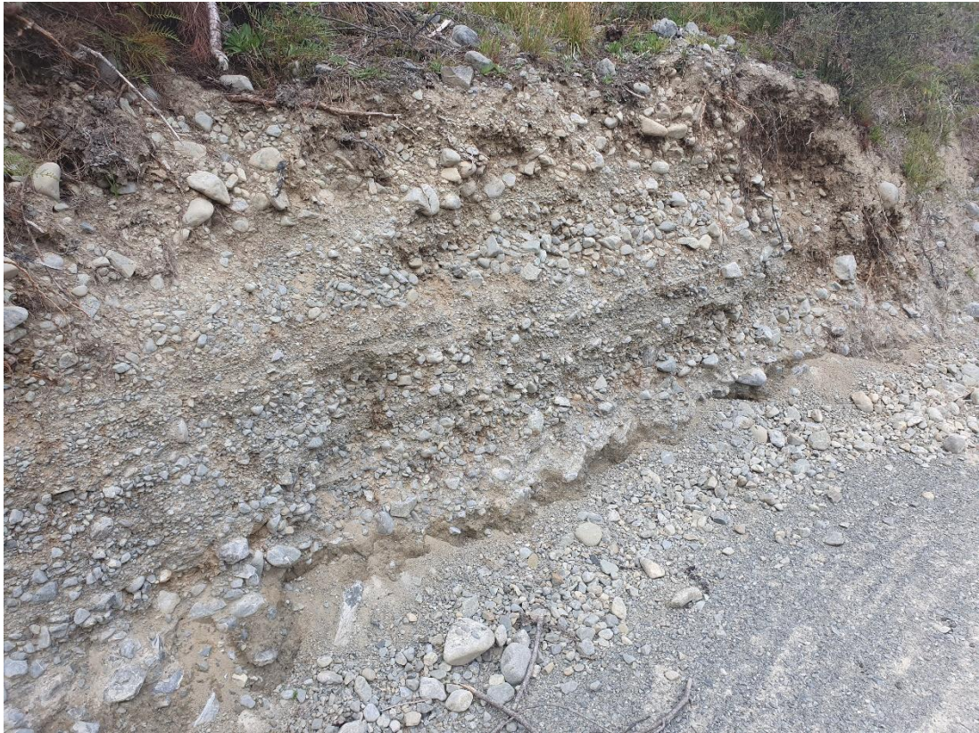
Figure 3 Exposure of the geology near to the Tasman Delta. Photo taken just west of Braemar Mount Cook Station Road, along one of the cuttings for the Alps to Ocean cycleway
