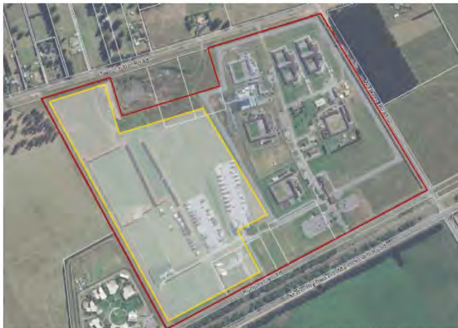
Figure 7: Aerial image of proposed 25 hectare assessment area at Rolleston Prison (yellow outline). Source: Boffa Miskell Limited.
