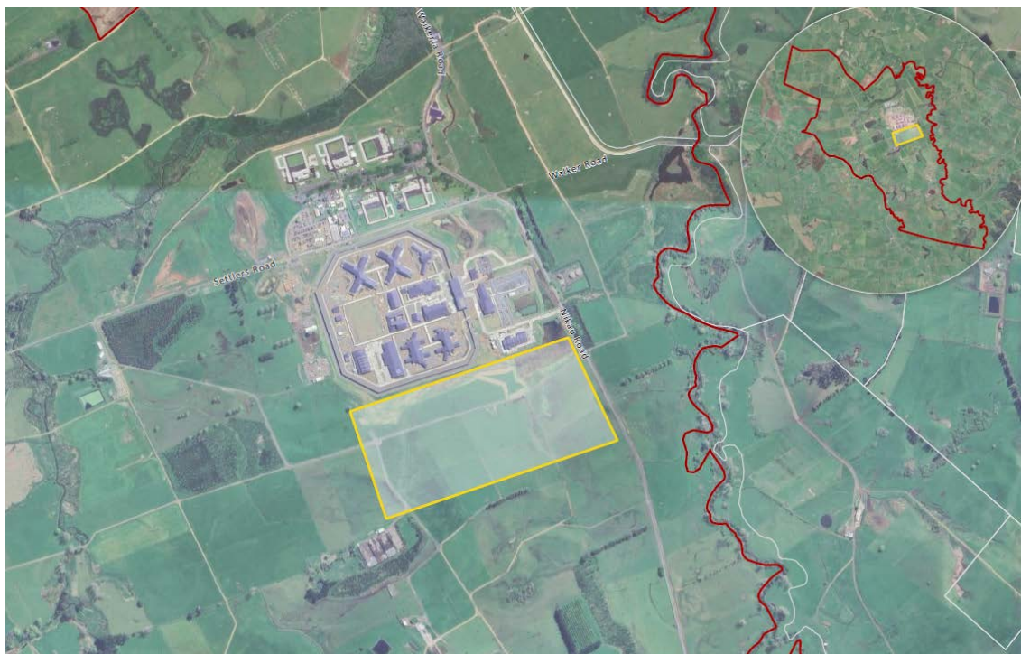
Figure 2: Waikeria Prison location plan. Prison Designation Boundary (red) Assessment Area 25 ha (Yellow).
