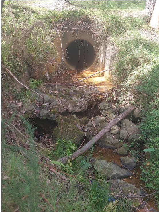
Upstream (eastern end) perched culvert
