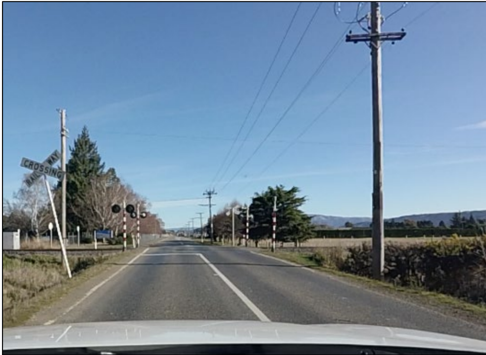
Photograph 3-9: Dukes Road North rail level crossing
