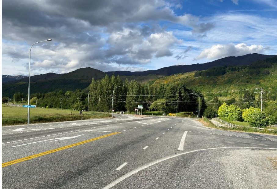
Photograph 5: State Highway 6 / Arrow Junction Road Intersection
