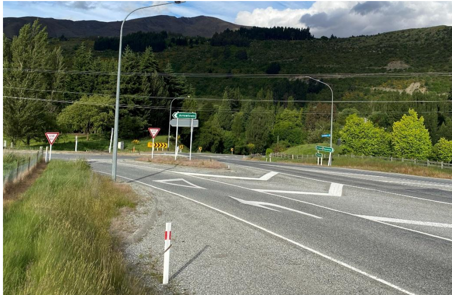
Photograph 6: State Highway 6 / McDonnell Road Intersection
