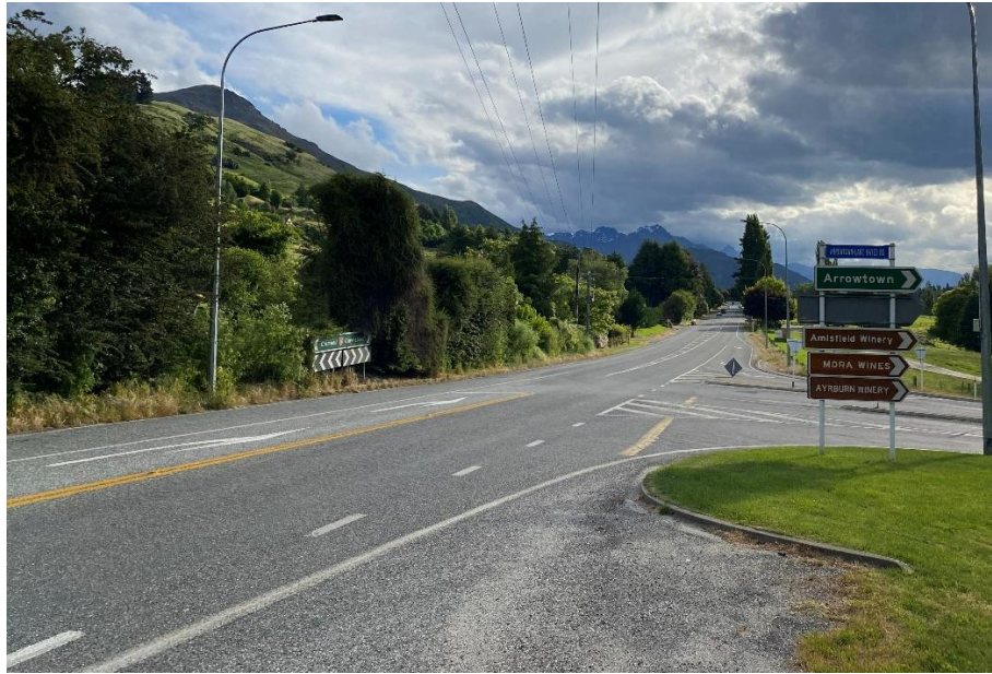
Photograph 3: State Highway 6 / Arrowtown Lake Hayes Road Intersection
