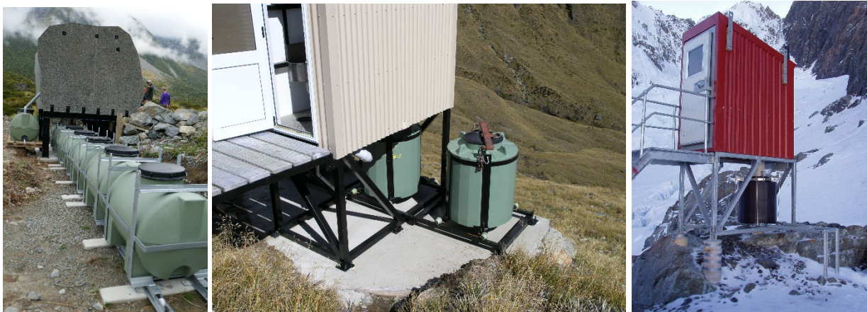
Figure 18. Examples of alpine drum containment toilets.
