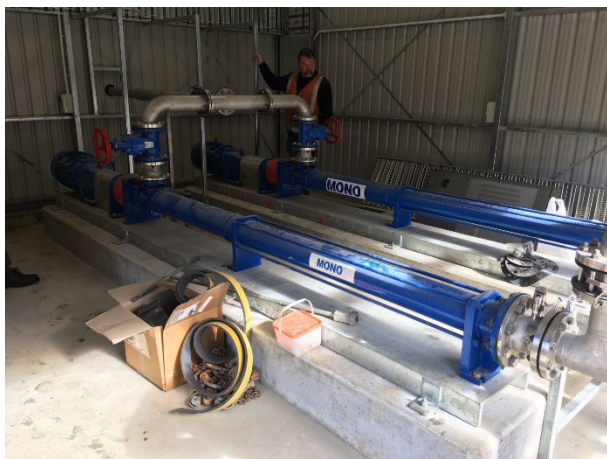
Figure 8. Example progressive cavity pumps
