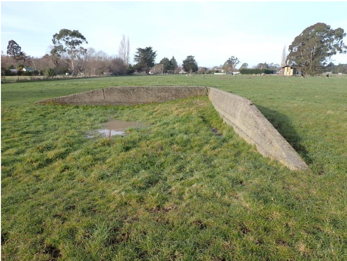
Figure 7-8. Internal view of concrete structure.
