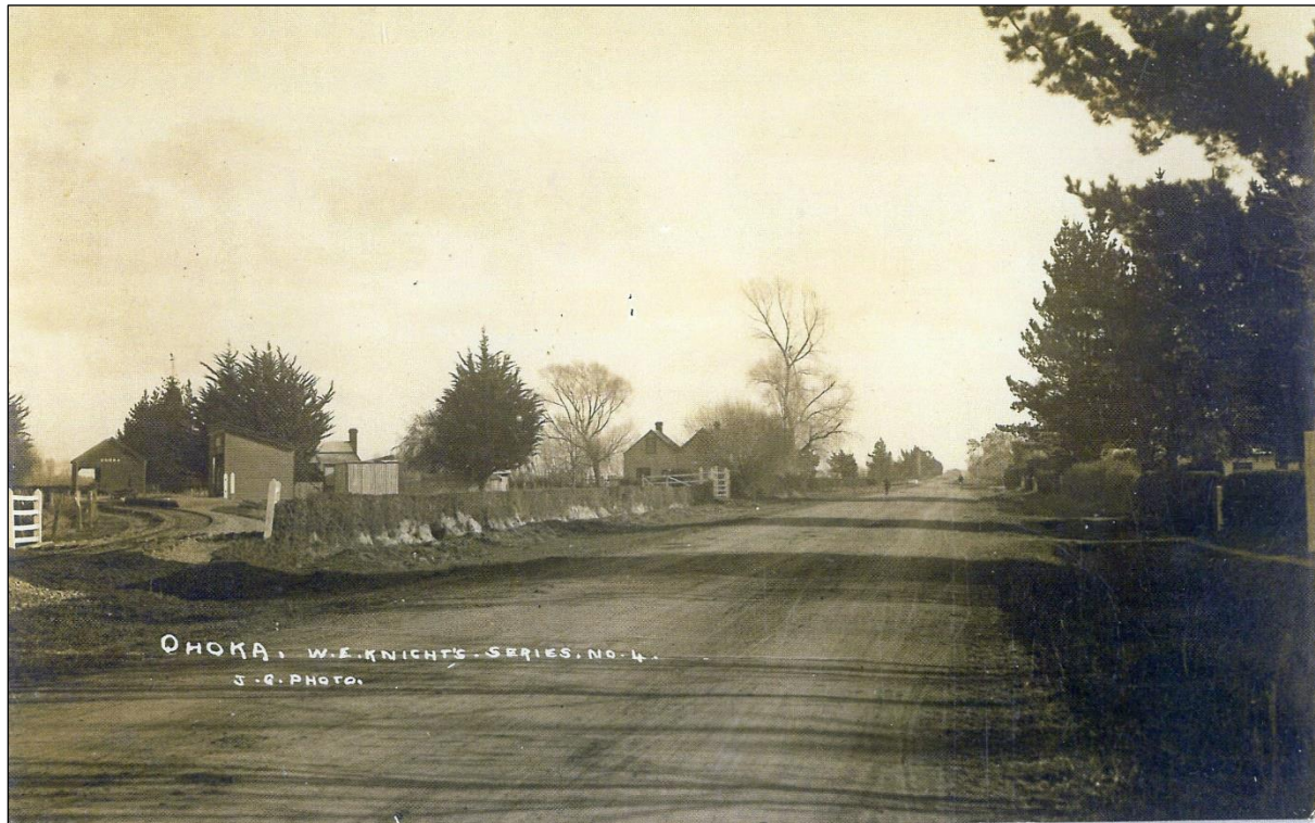
Figure 5-3. View of Mill Road looking west towards the Bradley Road intersection, with no specific date, but likely early 20 th century. A two-storied dwelling is visible at the centre of the image, which was the first Methodist parsonage. Image: Knight, n.d.
