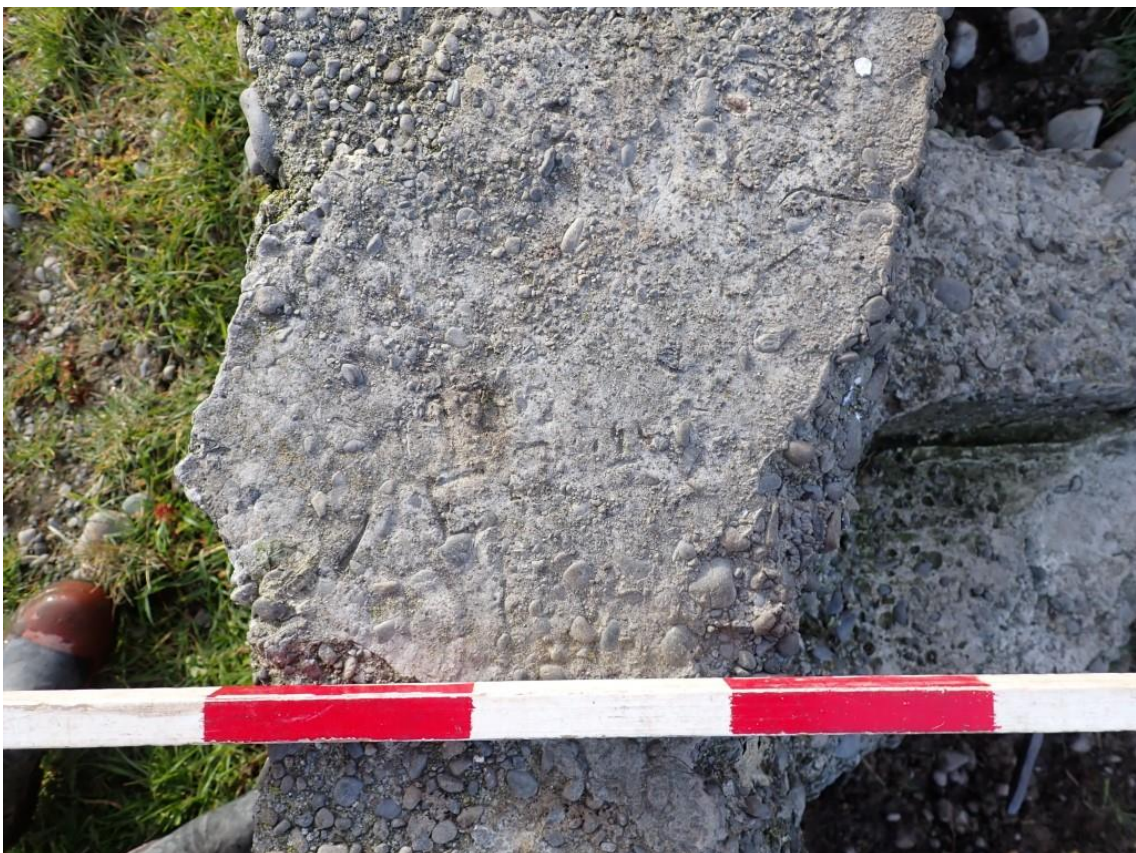
Figure 7-10. Possible marking/graffiti on concrete surface.
