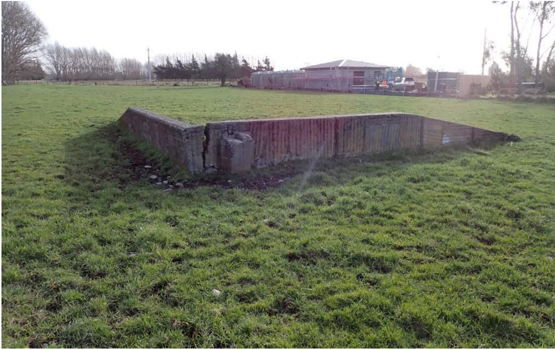
Figure 7-5. View of concrete structure within M35/1875.
