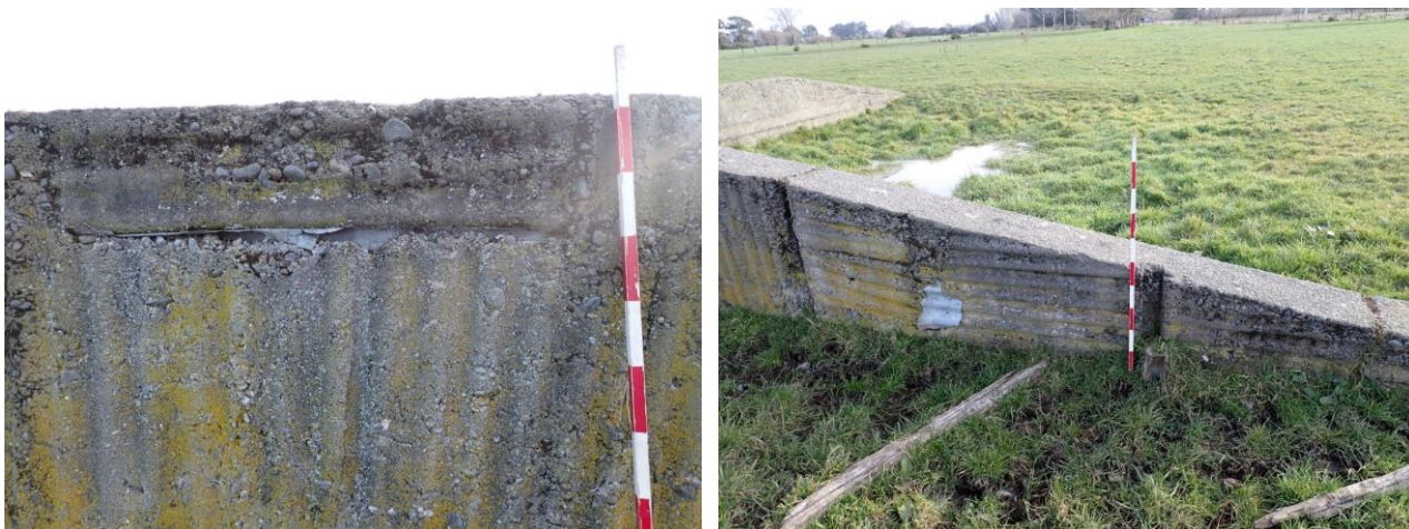
Figure 7-12. In situ corrugated iron and railway iron within northeast side.
