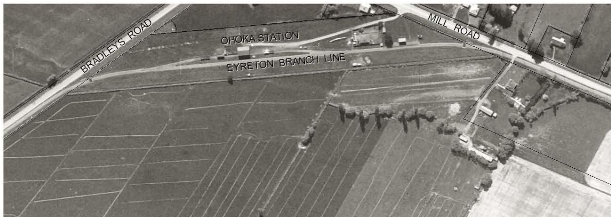
1940s aerial mapping photograph showing the Ohoka railway station.
