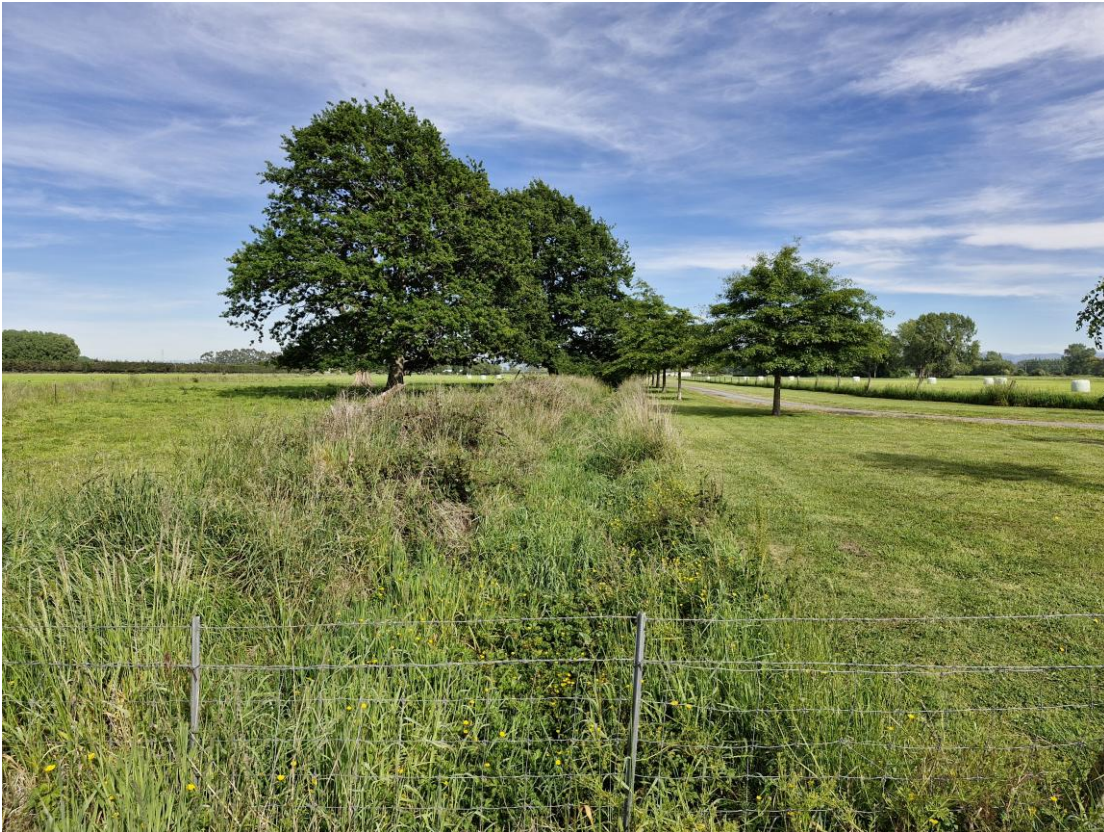
Figure 21: Unnamed Drain 2 at Whites Road
