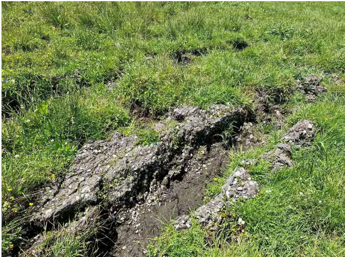
Photograph 8: Vehicle tracks in wet soils near Wetland 8. Surface cracking indicates the disturbance was not recent, 535 Mill Road.
