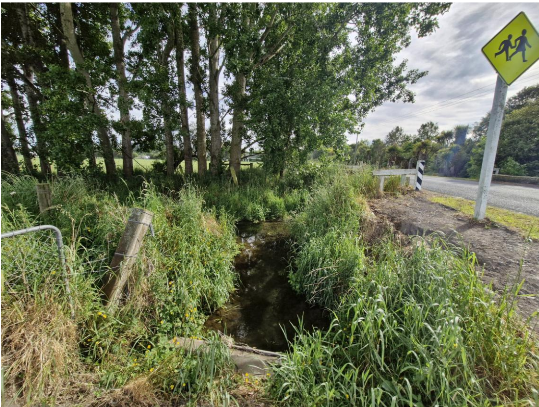
Figure 6: Whites Road Drain, view northeast at Ōhoka Stream Tributary confluence.
