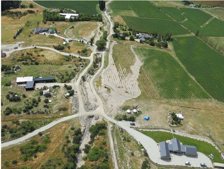
Fig. 13: Aerial view looking down the fan and channel. The 1 st culvert is in the foreground. Finer grained flows which escaped the channel travelled a long distance down the fan surface
