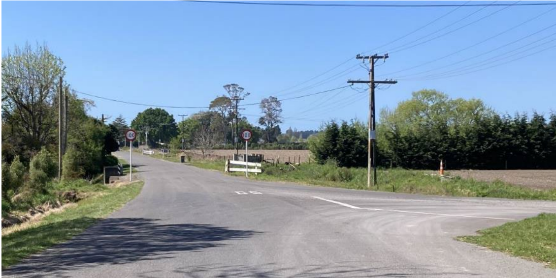
FIGURE 4 – BROOKVALE ROAD LOOKING EAST TOWARDS SITE ACCESS (ON RIGHT)
