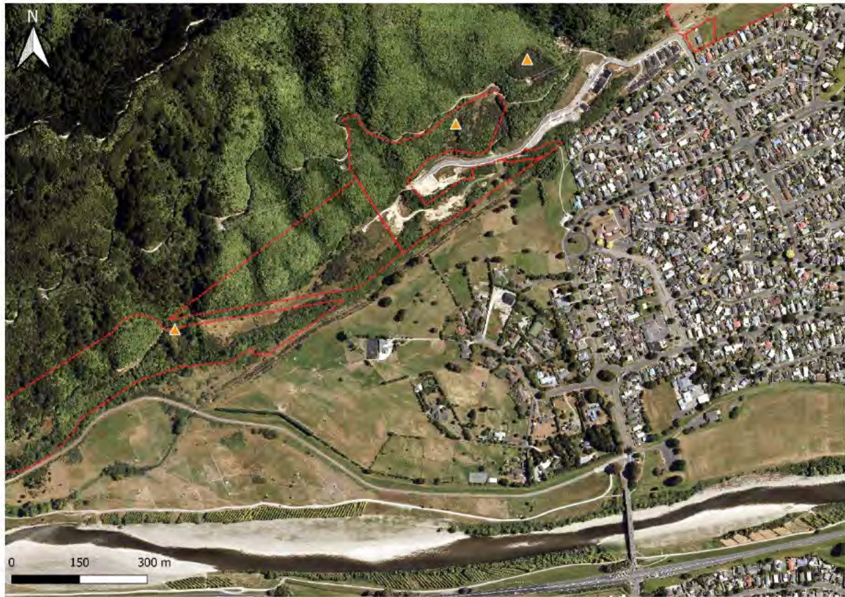
Figure 4: Recorded Landslides in the New Zealand Landslide Database.
