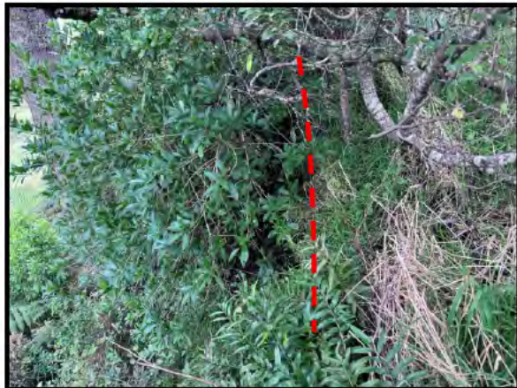
Photo 8: Small-scale failure at terrace crest (red dashed line).
