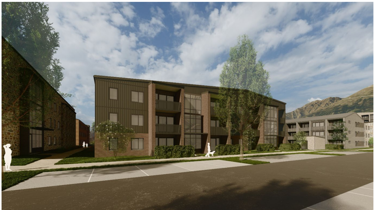
Figure 07: Metal cladding on upper two floors of Building 3 looking from Road 01.
