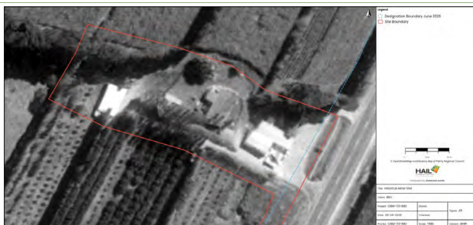
1992 - Large shed erected in west of site, and large shed in the east.
