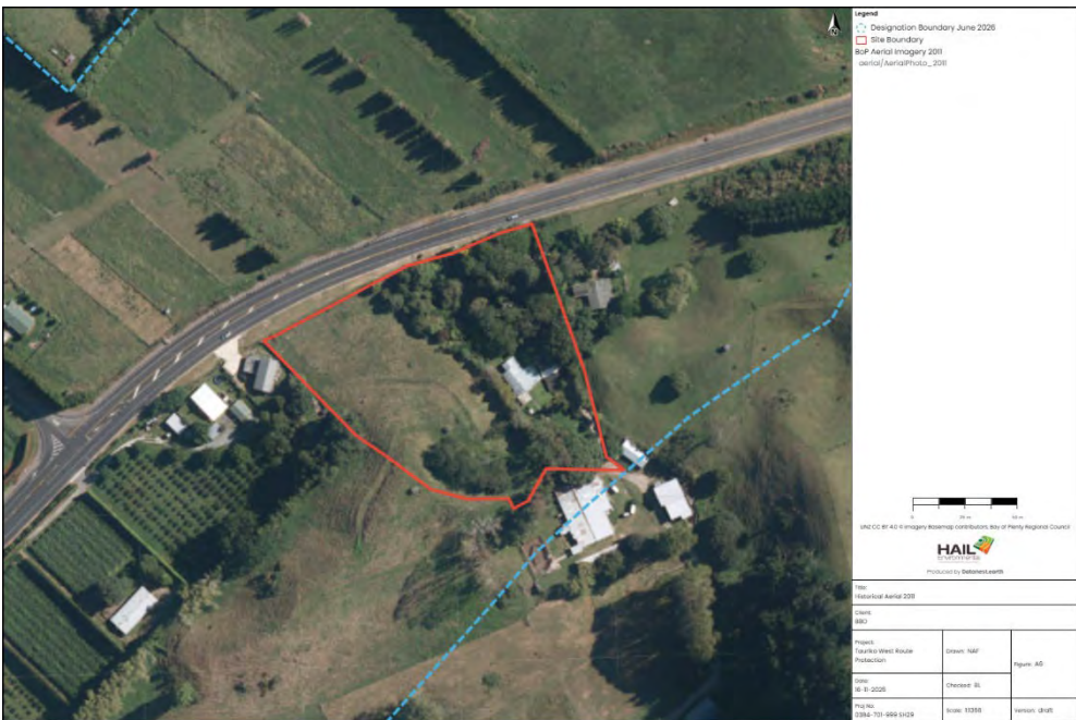
2011 - Building appears to be residential, clothesline in backyard.
