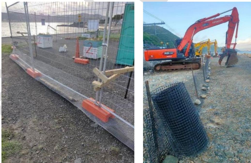
Figure 7: Examples of fencing to exclude kororā from work areas
