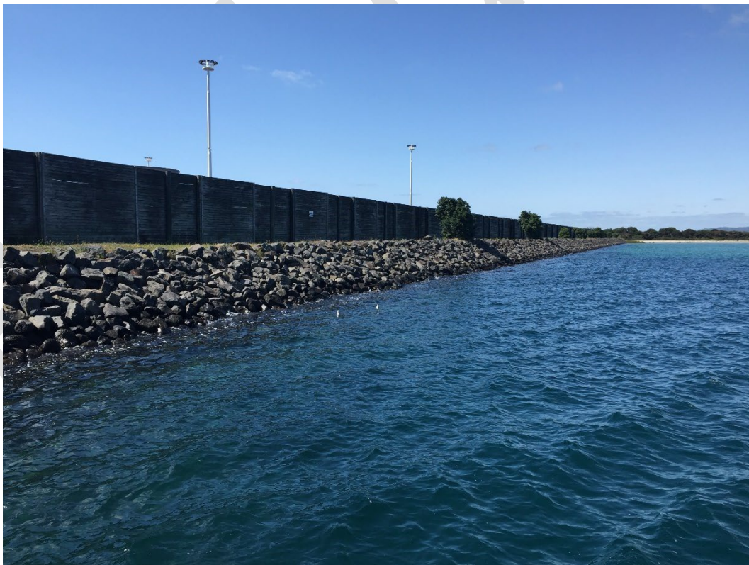
Photo 3: Potential kororā habitat within the riprap revetment along Northport western boundary
