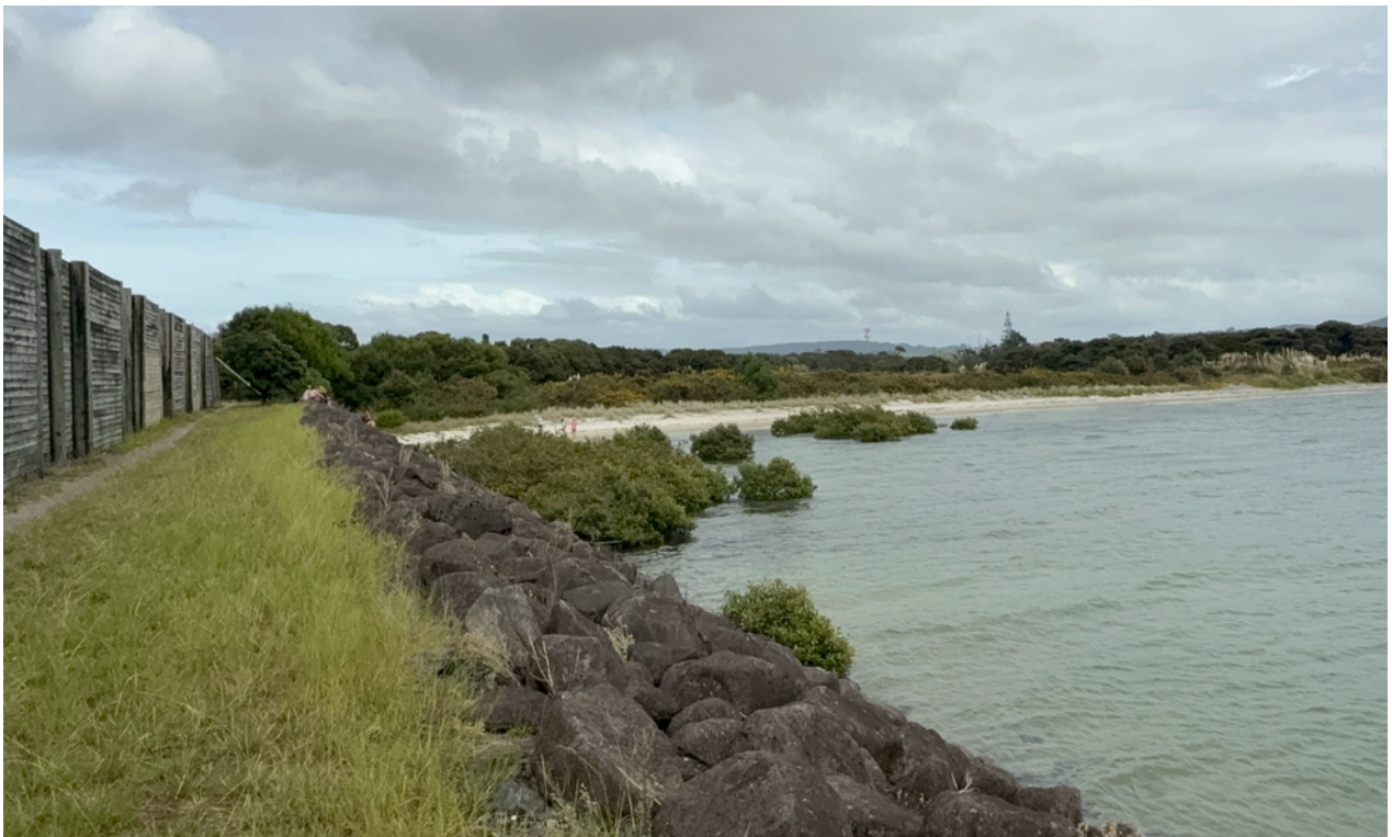
Figure 25 Beach looking south from existing revetment wall
