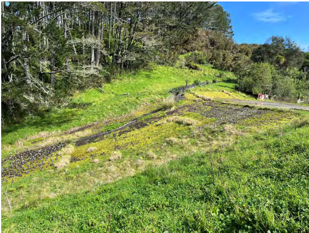
Photo 7 – Pond 5 spillway vegetated with moss and some grasses, looking west.
