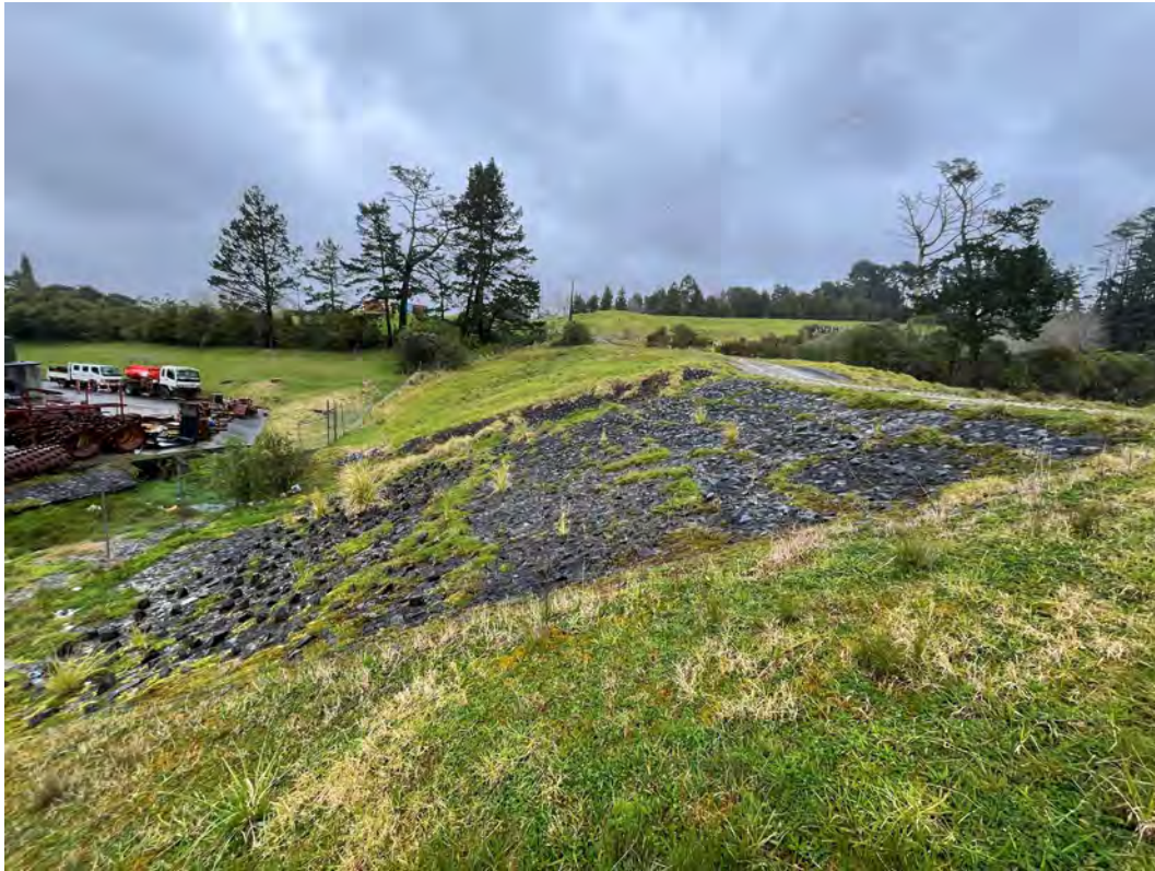
Photo 14 – Pond 6 spillway with some minor vegetation, looking south.
