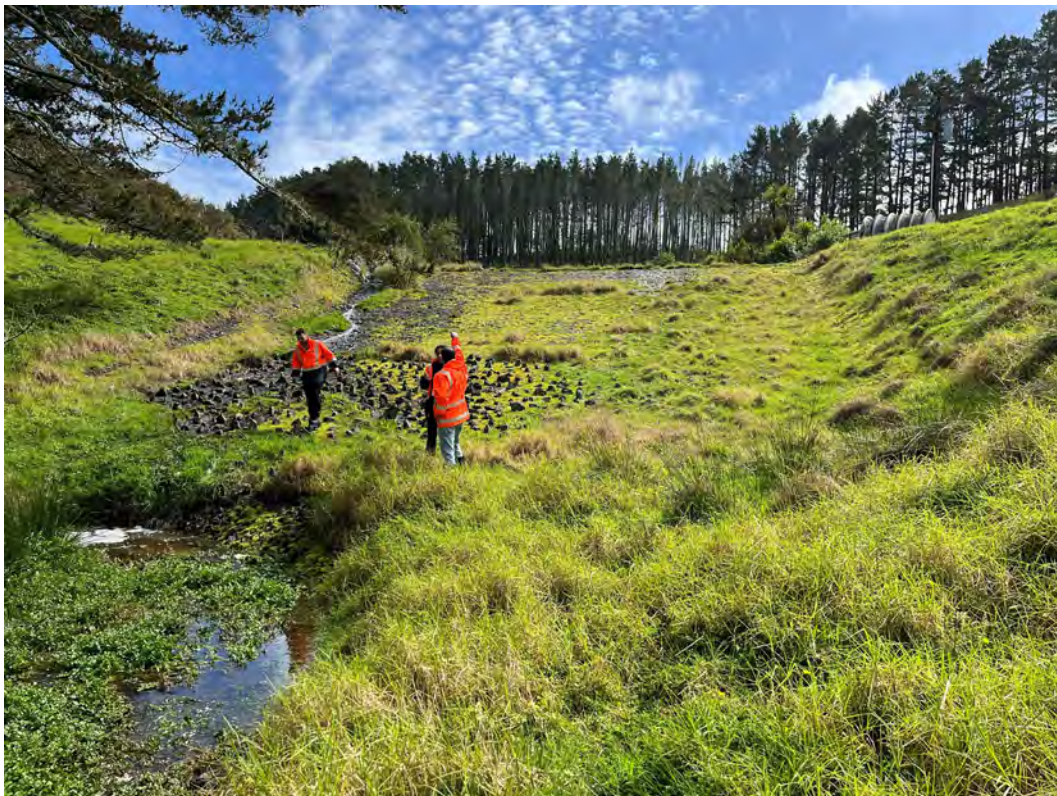
Photo 9 – Pond 5 spillway looking north, ponded water at base of spillway.
