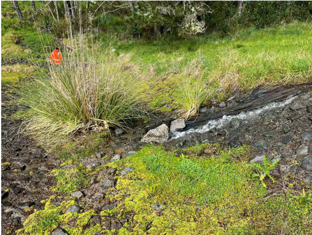
Photo 8 – Outlet of clean water diversion onto the Pond 5 spillway.
