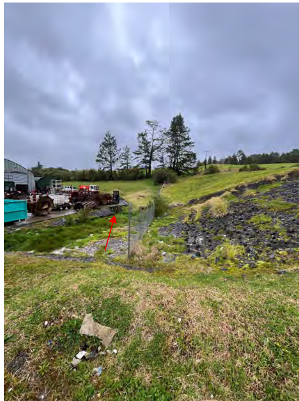
Photo 15 – Pond 6 spillway, looking south, ponded water at base (LHS of fence) draining out the culvert (marked with arrow).
