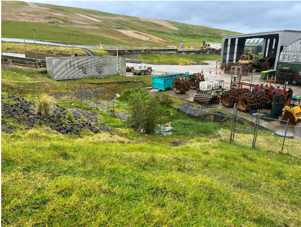
Photo 16 – Bottom of Pond 6 spillway, looking northeast.
