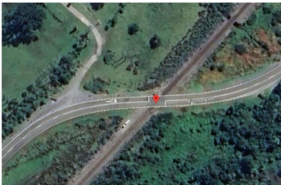
Figure 3-2: SH67 Kerrs Road Granity level crossing aerial (Source: Google Maps)
