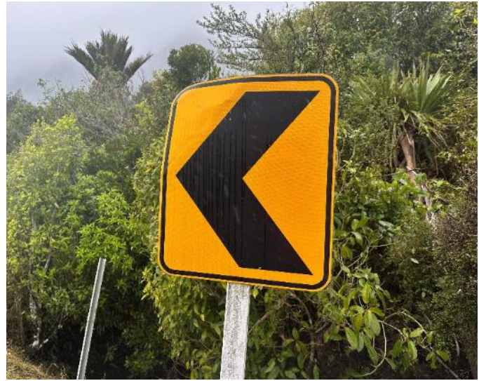
Figure 3-19: Damaged single chevron sign
