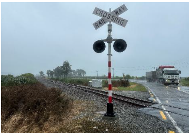
Figure 3-7: DOWN track sightline on northern approach
