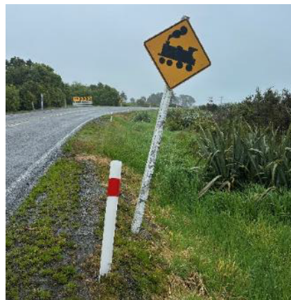
Figure 3-15: WX1R sign on northern approach is damaged.
