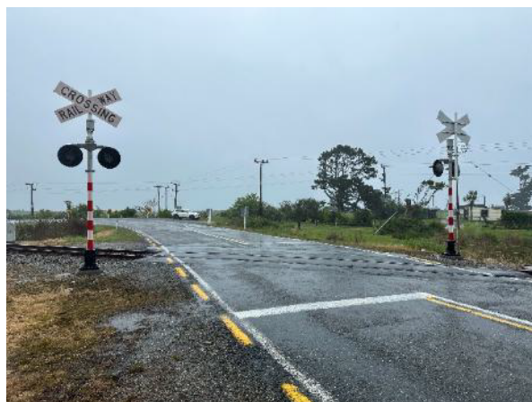
Figure 3-4: Northern approach to the level crossing from Birchfield Road
