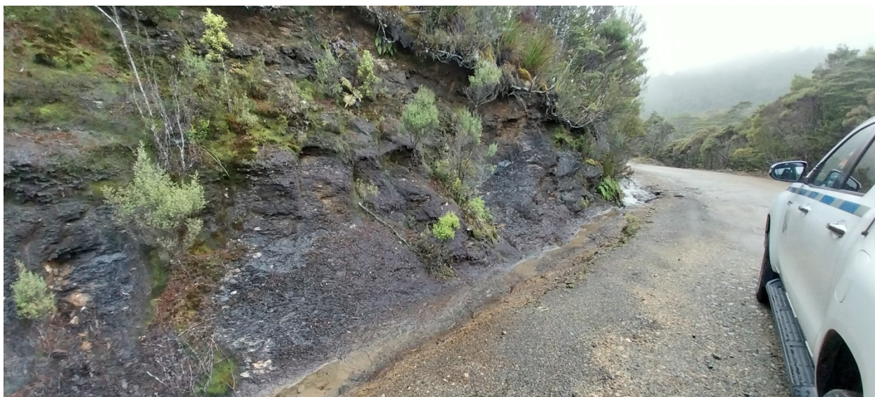
Figure 6: Kaiata Mudstone Cutting along haul road alignment
