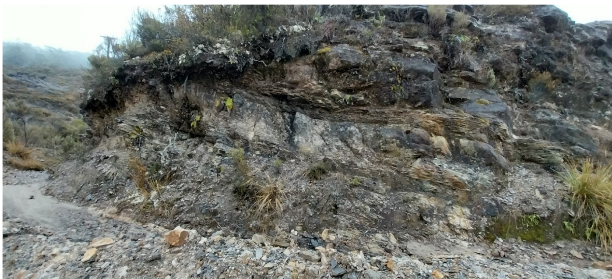
Figure 7: Brunner Coal Measures cutting on haul road alignment
