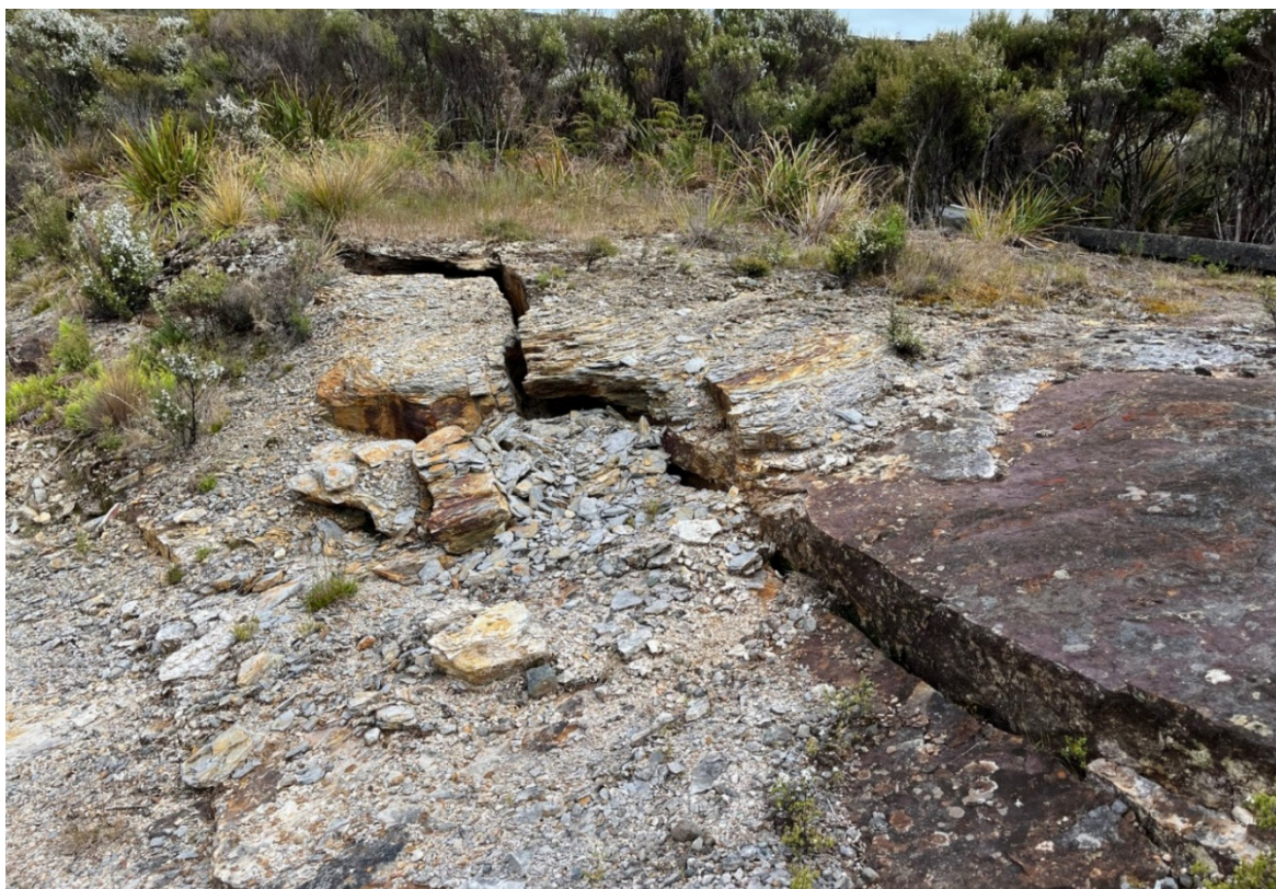
Figure 14: Surface cracking above Iron Bridge historic mine. Location of image is depicted as (1) on Figure 5.
