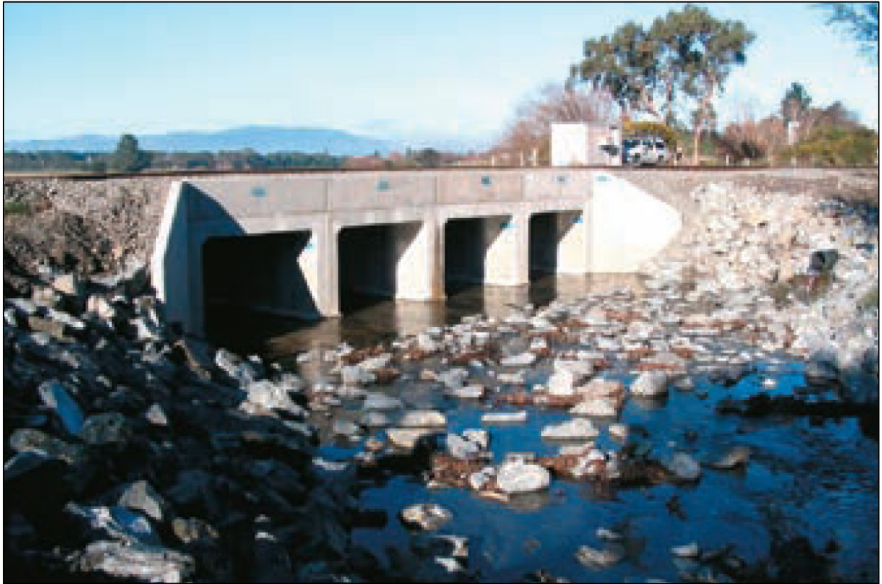
Figure 26: Box Culvert Installation similar in geometry to that proposed
