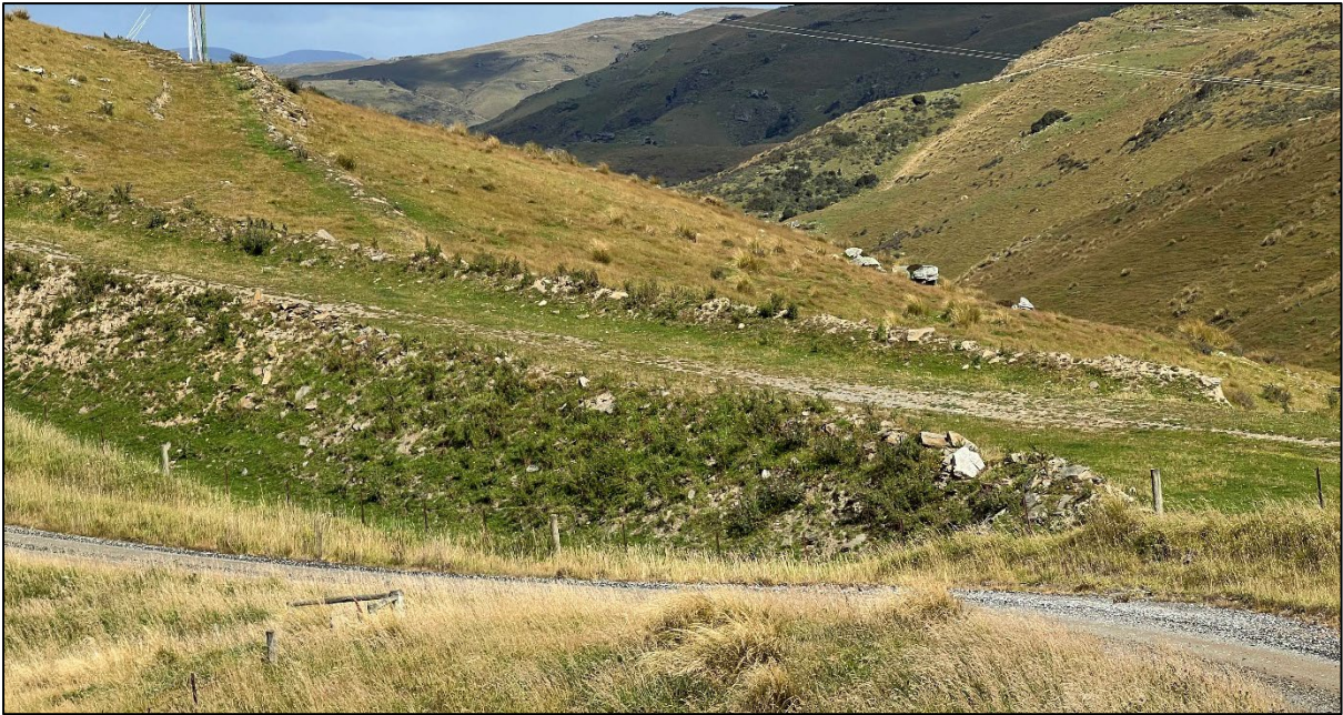
Figure 133. Example of the existing haul road formation, with Golden Bar Road in the foreground.
