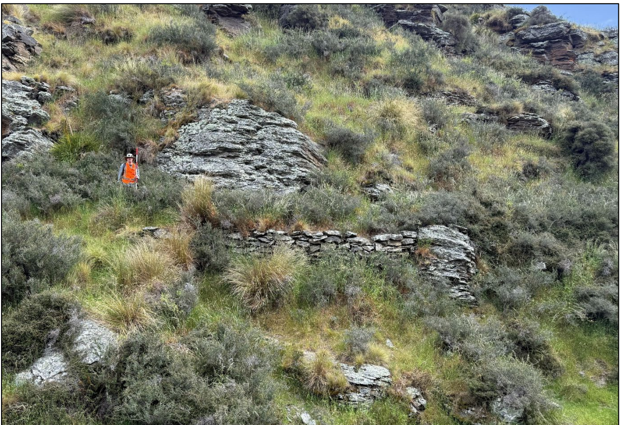
Figure 155. Further revetment on west slope of gully (CC05).
