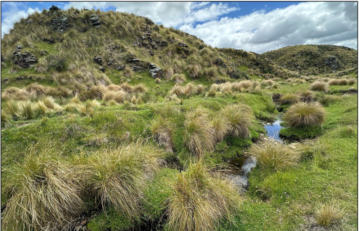
Figure 184. Earthen mound of the tram causeway running north to south (CC14), looking east.
