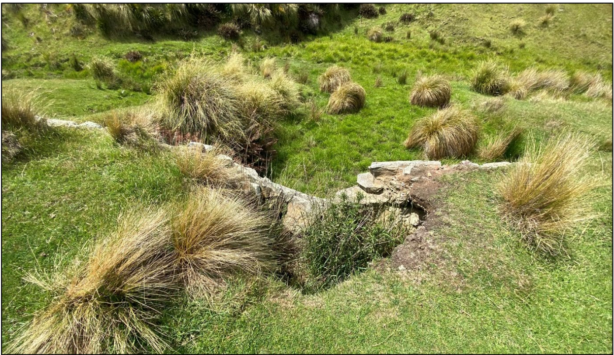
Figure 115. Plan view of collapsed area in major revetement along track/road (previous two photographs), looking north-east.
