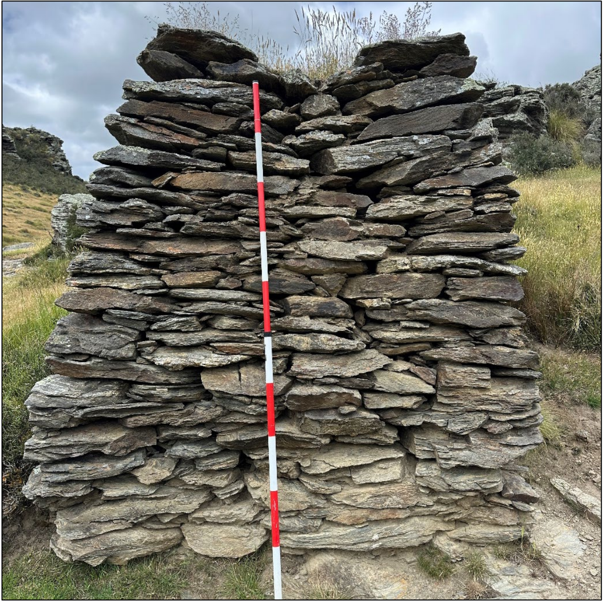
Figure 162. Large revetment with notable curve in the top centre, possibly to accommodate a flume, looking south (CC10).
