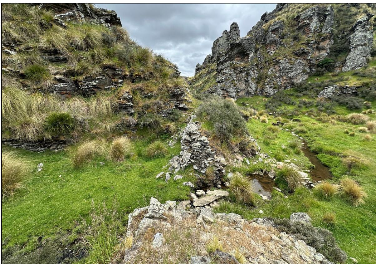
Figure 161. Breached revetment, looking north (CC09).
