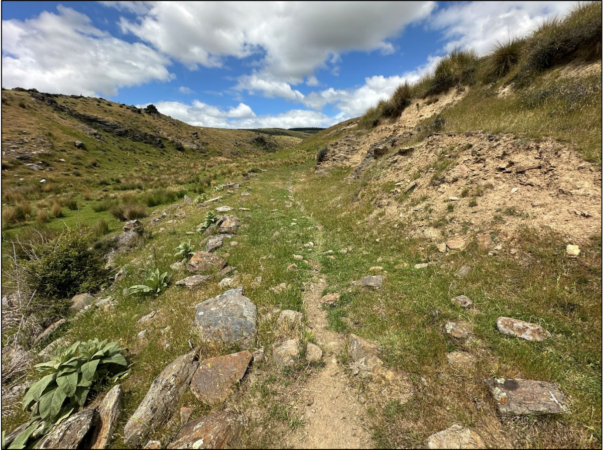
Figure 189. Cutting from hillside for the tramway (CC18), looking south.
