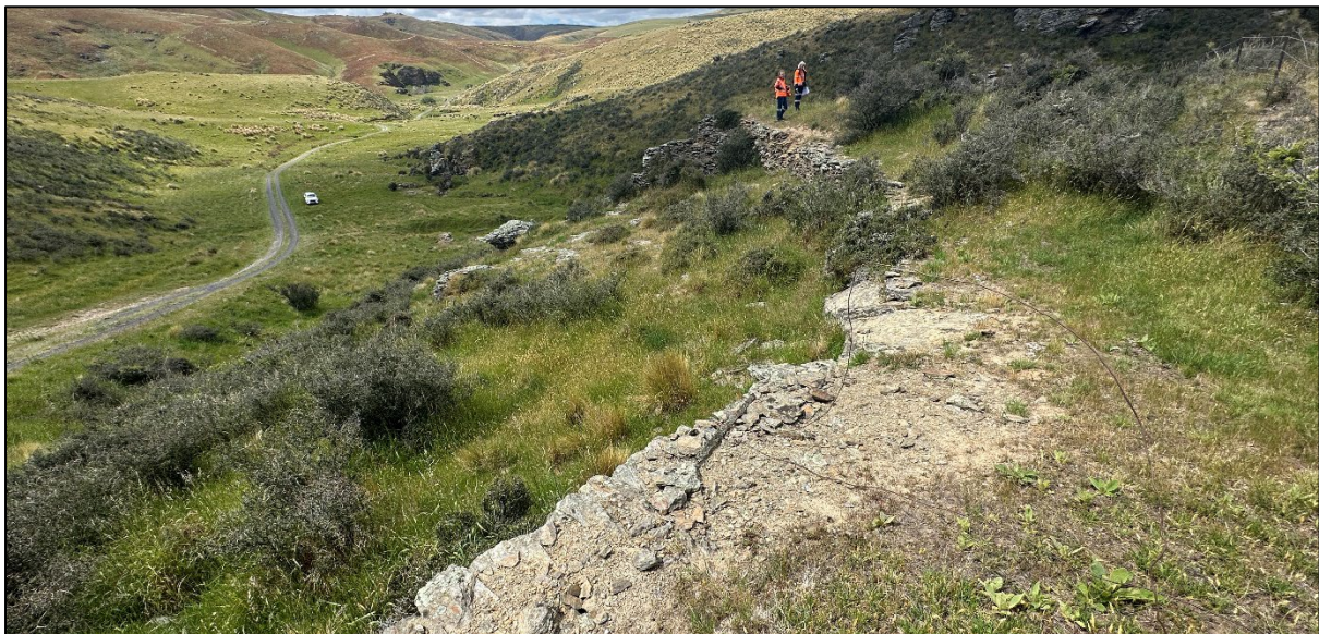
Figure 149. Revetment (CC01), at far north near battery location, looking east.
