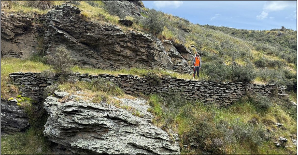
Figure 154. Revetment on the western slope of the gully within the dam footprint (CC04), looking west.
