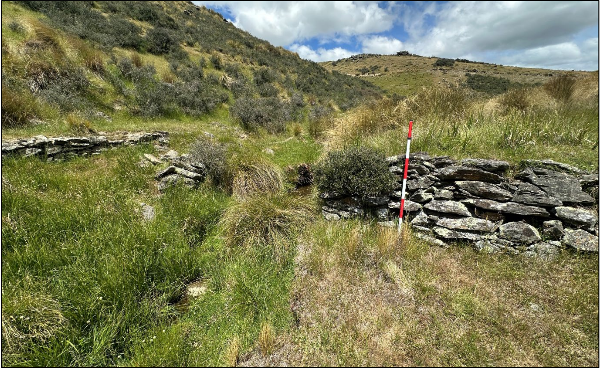
Figure 175. Photo of C24 and C25 showing collapsed portion of C24 revetment that once abutted CC25.
