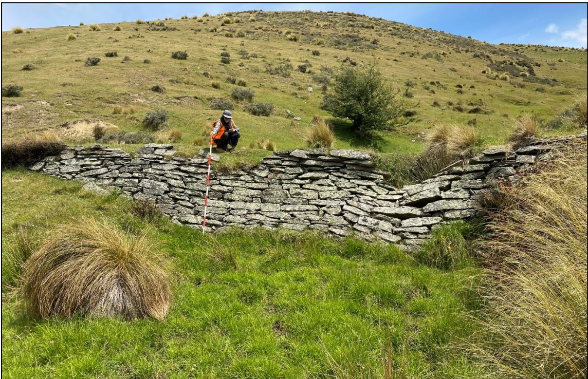
Figure 113. Major revetment along track, looking south-west.
