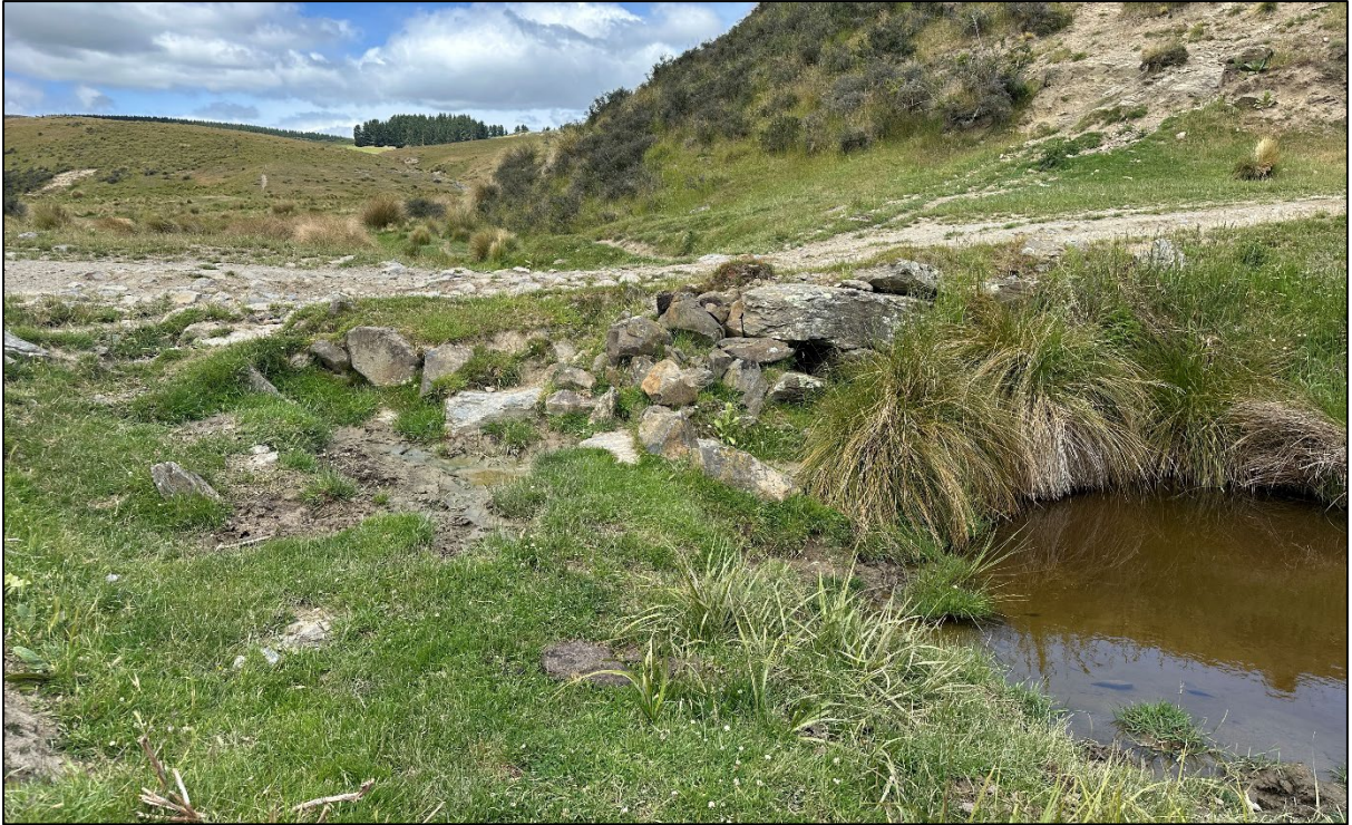
Figure 179. Remains of stone revetment that once crossed the stream (CC21).
