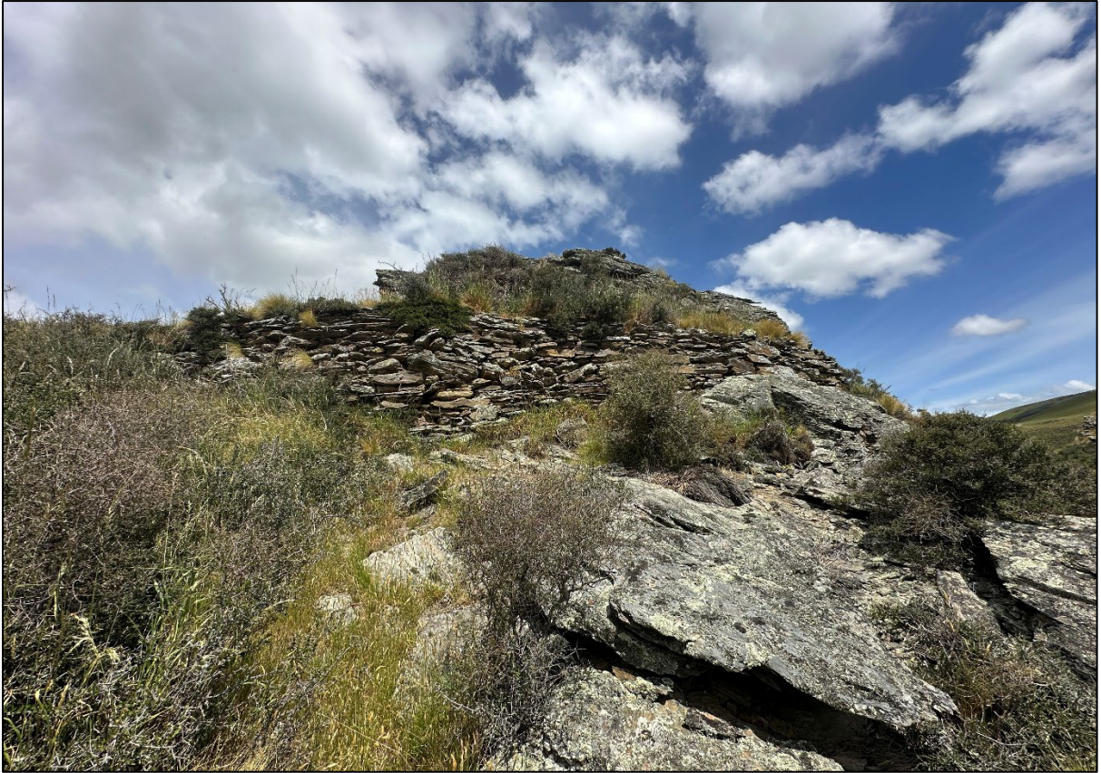
Figure 156. Revetment identified at high elevation outcropping on eastern side of gorge (CC06, CC07), looks south.
