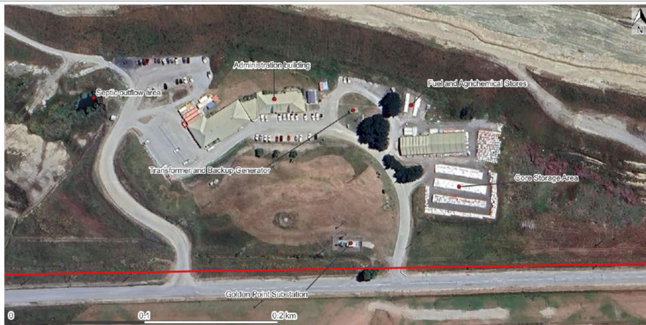
Figure 14. Golden point substation and administration building location (image source: Google Earth)
