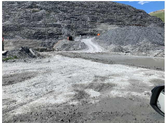
Photograph 5. Concrete washings at the Golden Point portal
