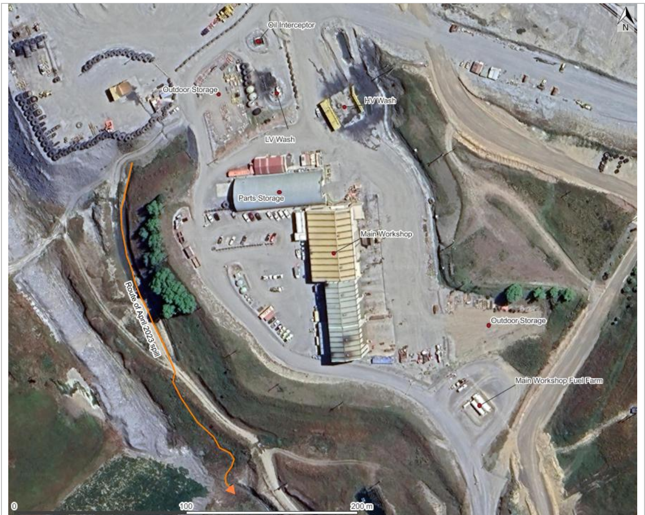
Figure 11. Main open pit workshop and surrounds (image source: Google Earth). Spill route shown as orange line
