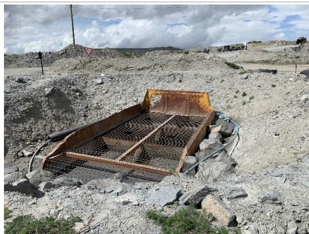
Photograph 17. Oil-water separator for both vehicle washes
