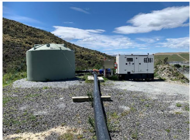
Photograph 33. Typical pumping station set up
