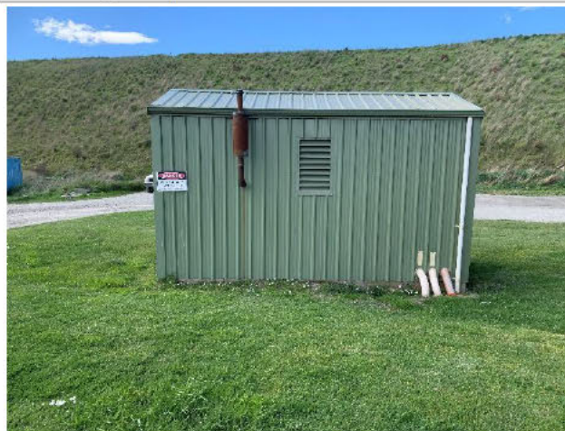
Photograph 30. Backup generator building next to main office
