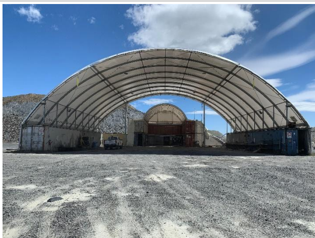
Photograph 7. Former Coronation Workshop
