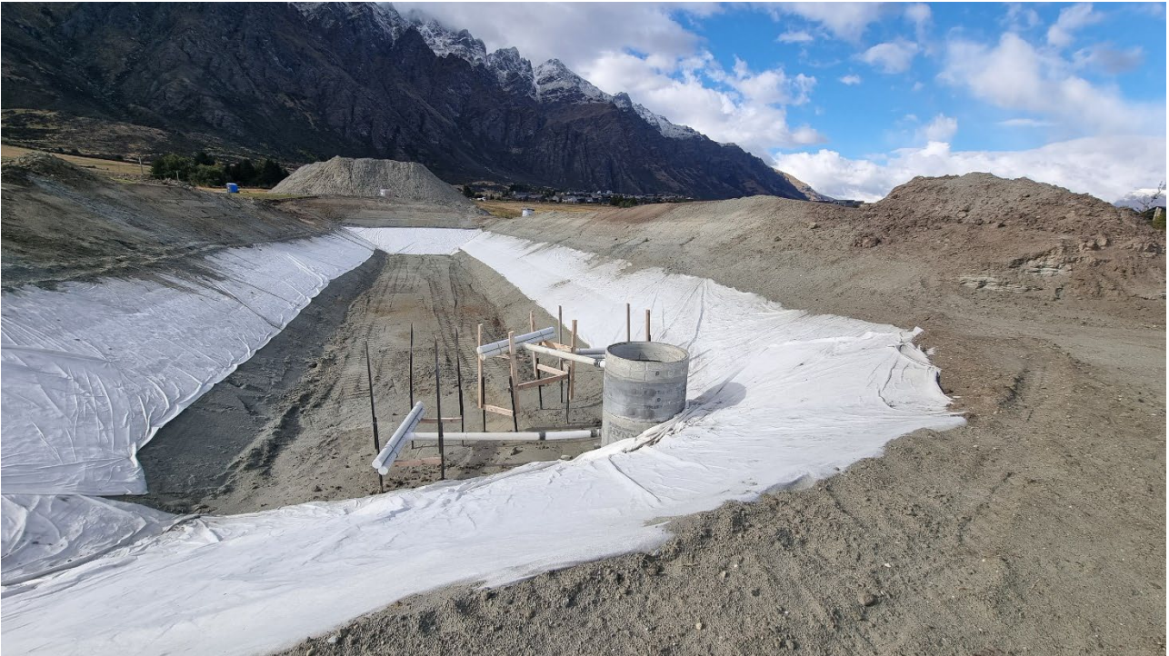
Figure 6-5: Sediment Retention Pond outlet example
