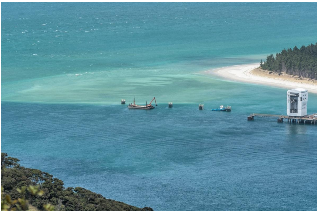
A photo of backhoe dredging occurring off Marsden Point in March 2017, taken from Mt Aubrey
