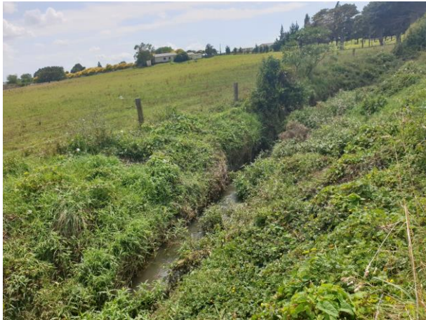
Photo 32. Watercourse 3 had been modified through straightening and deepening.
