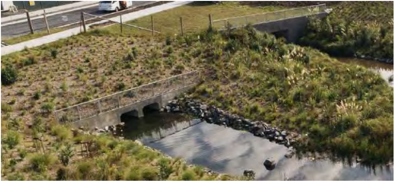
Figure 19 Culvert headwall/wingwalls
