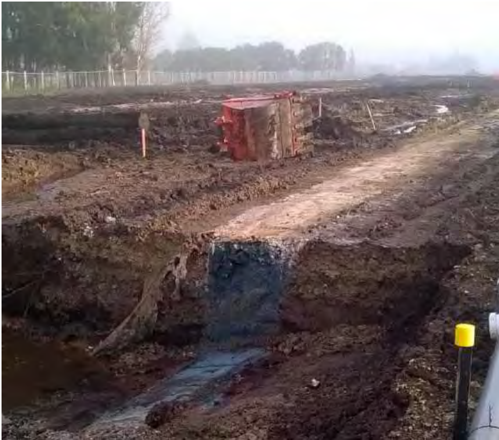
Figure 20 Slurry wall photo
