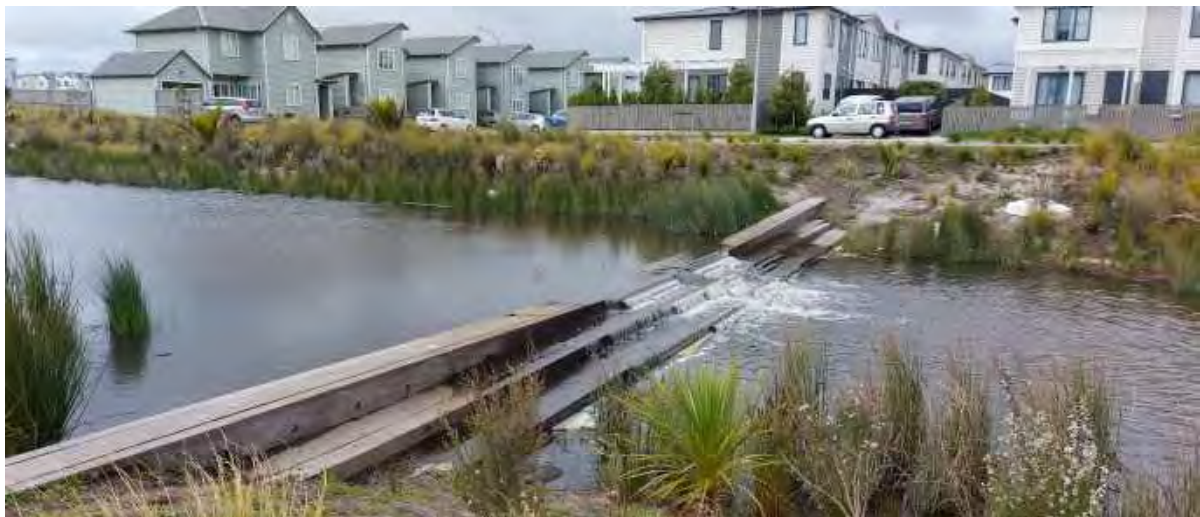
Figure 15 Photo of weirs from Awakeri Wetlands Stage 1
