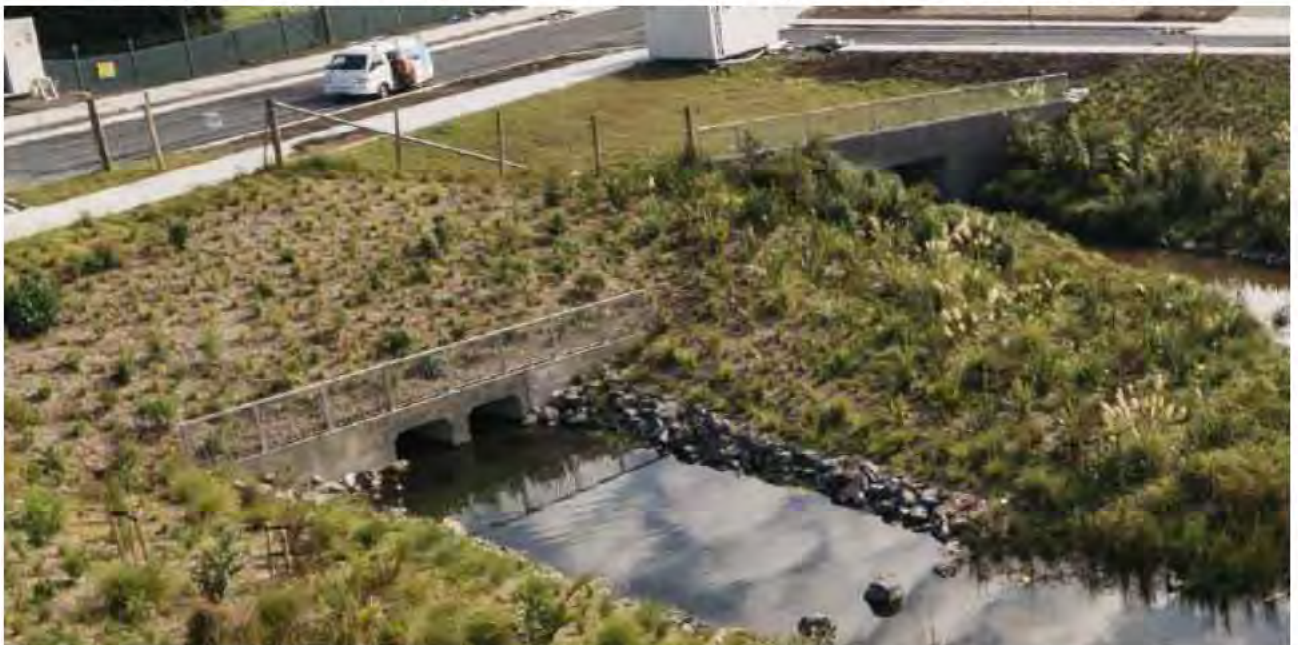
Figure 2 Culvert headwall/wingwalls
