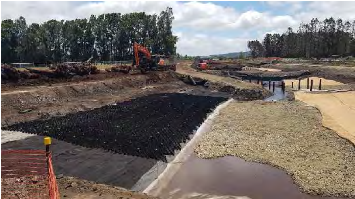
Figure 4 Geoweb scour protection, enkat and gravel lining for underwater wetland base
