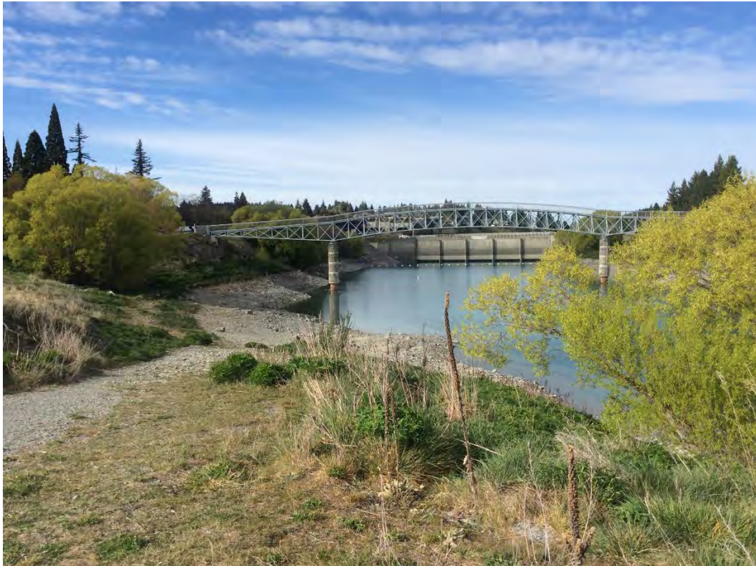
Photo 4: Takapō River control gate survey location.
