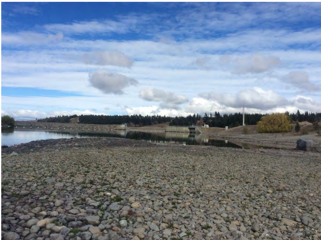
Photo 5: Canal gate survey location.
