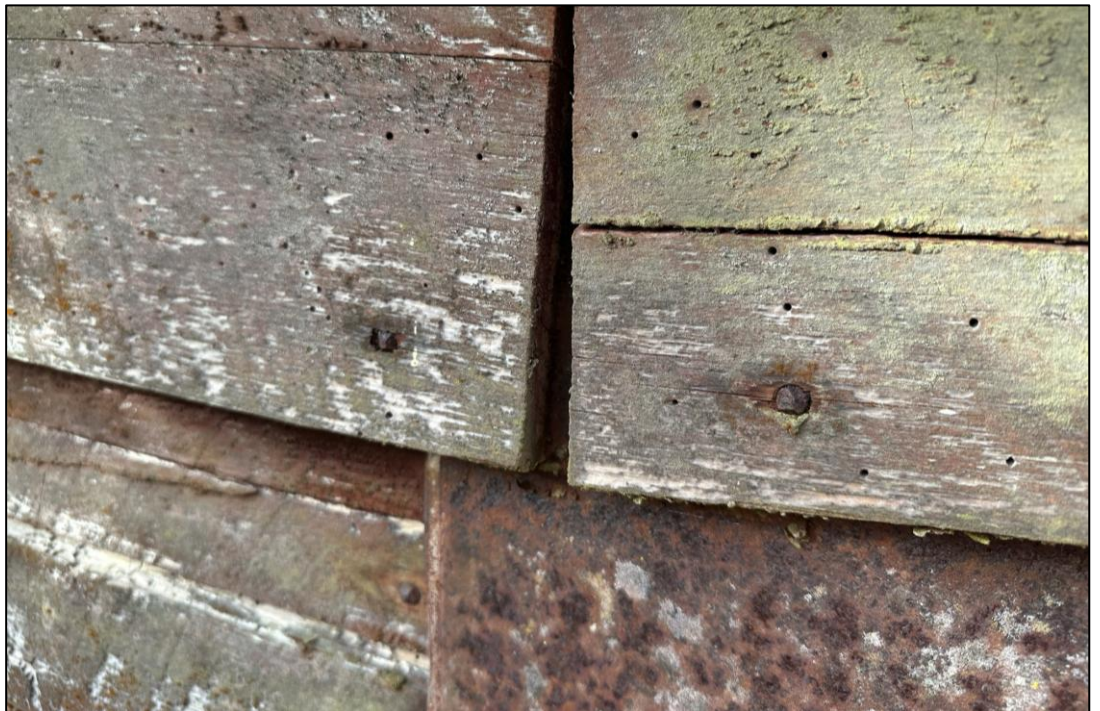
Figure 19 Close up of weatherboards and nails.
