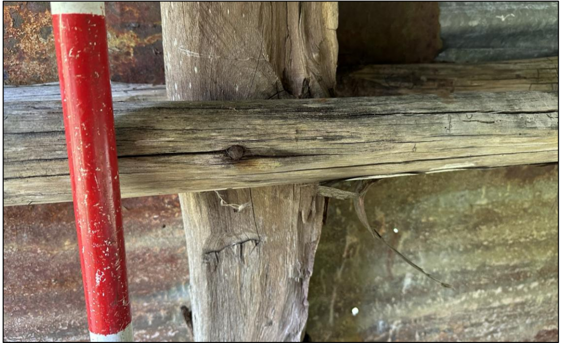
Figure 27 Nail in framing of southeast wall.
