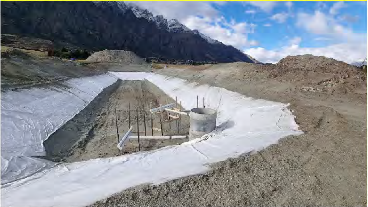
Figure 6-5: Sediment Retention Pond outlet example
