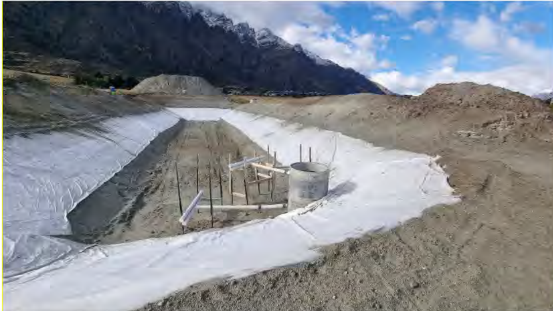
Figure 6-4: Sediment Retention Pond outlet example
