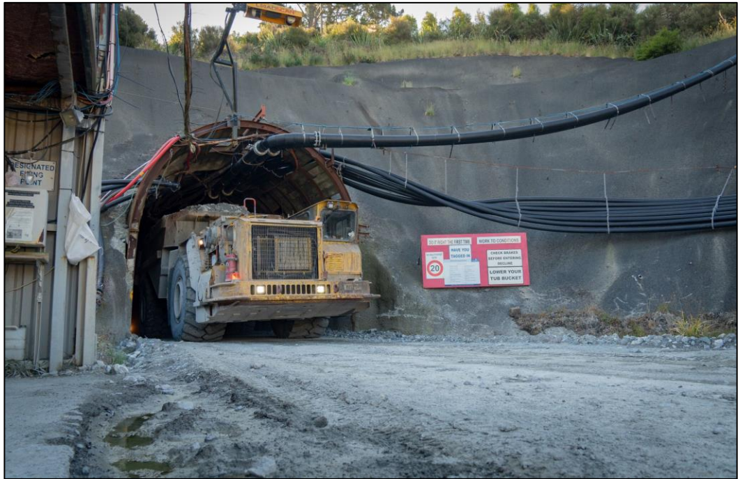
Figure 2-32: Example Access Tunnel Portal
