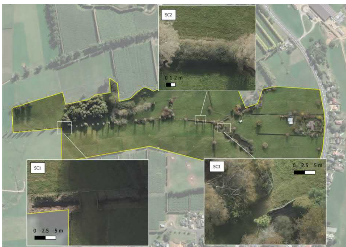
Figure 4.2: Locations of watercourse crossings (SC1, SC2, SC3).
