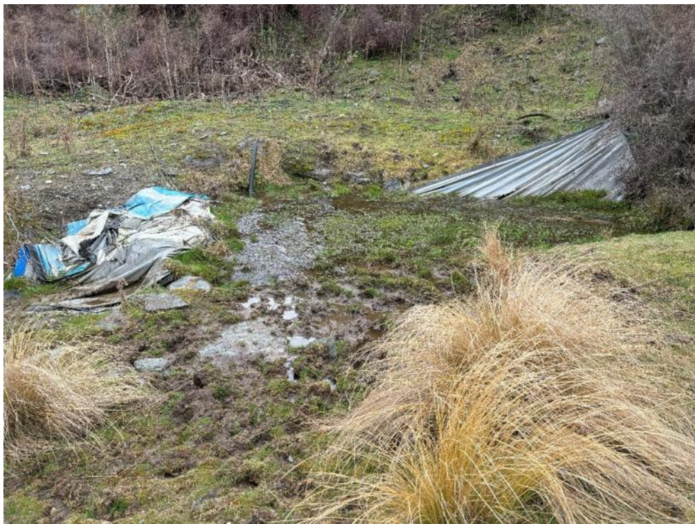
Figure 43: The stock water intake structure in Shepherds Creek.
