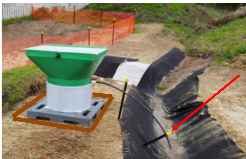
Figure 8 Example of Floc Box setup. Note discharge line staked in drip into the centre of the dirty water diversion
