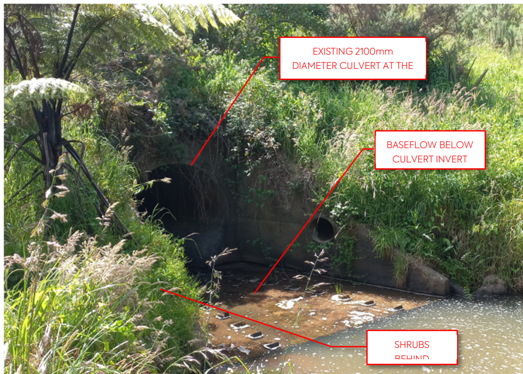
Figure 7 - Inlet of Culvert under State Highway 1
