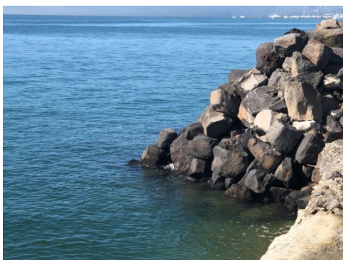
Figure 24. Upper: West end of Fergusson North berth showing Interface between end of existing eastern revetment and mudcrete reclamation.
