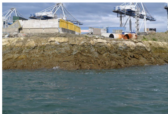
Figure 24. Upper: West end of Fergusson North berth showing Interface between end of existing eastern revetment and mudcrete reclamation.
