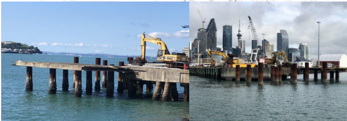
Figure 23: Piles and deck at north-east corner of Bledisloe Terminal to be demolished.
