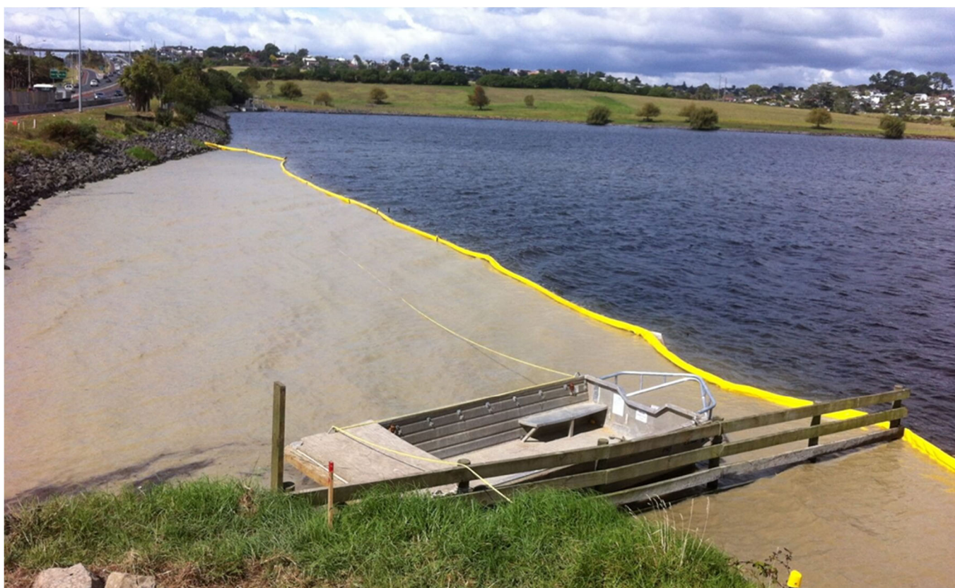
Figure 17 Example of floating sediment curtain ( https://cirtexcivil.co.nz/products/silt-control/envirosieve-turbidity-curtain/ )
