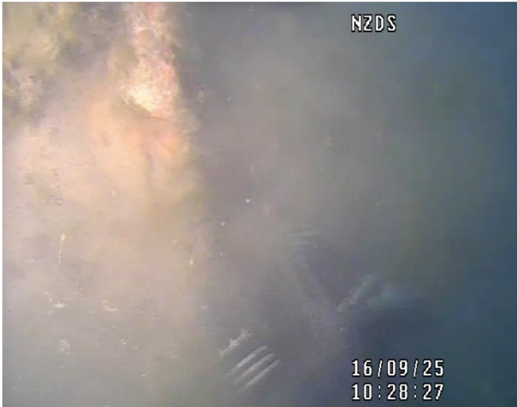
Figure 2-13. Example of exposed reinforcement on ribs (Rib 1).
