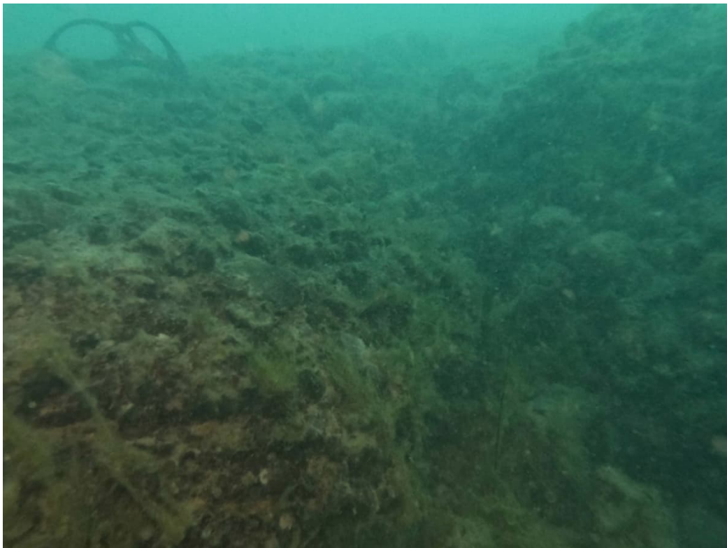
Figure 2-3. Example of channel formed in top surface of control weir.
