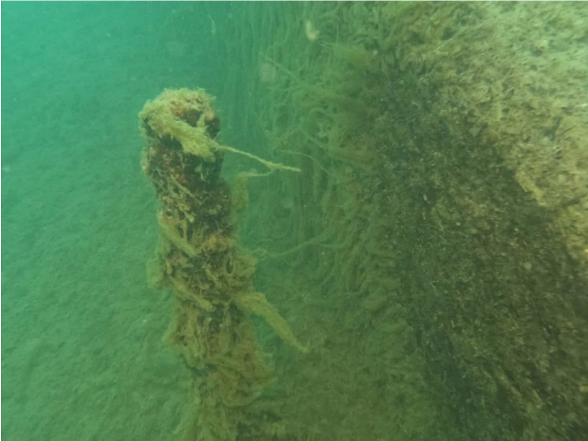
Figure 2-6. Example of exposed vertical reinforcement on control weir.
