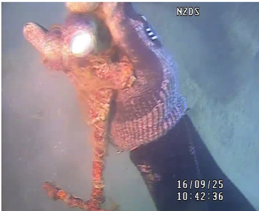
Figure 2-14. Loose mesh reinforcing on Rib 1.
