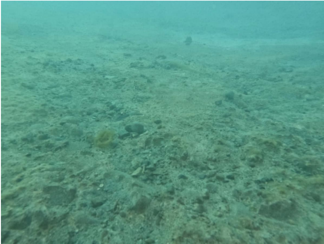
Figure 2-2. Picture of typical surface condition of control weir.
