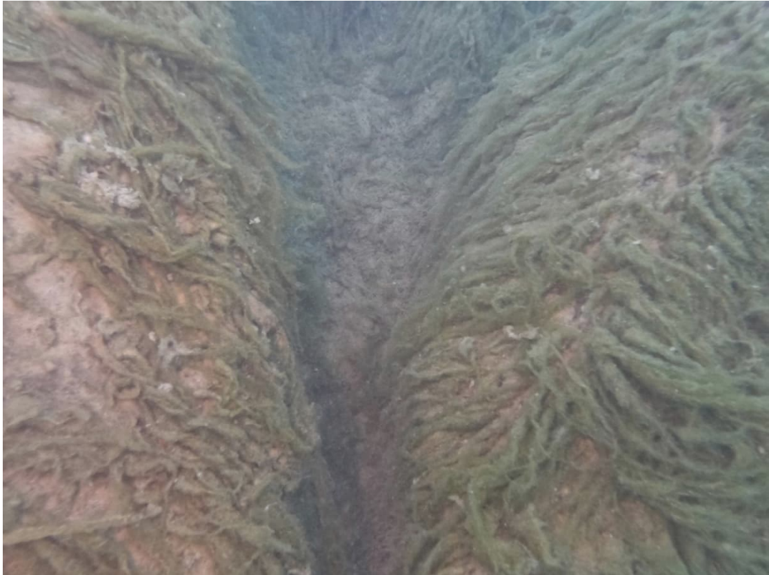
Figure 2-11. Example of V-shaped channel in concrete on top of rib surface (Rib 1).
