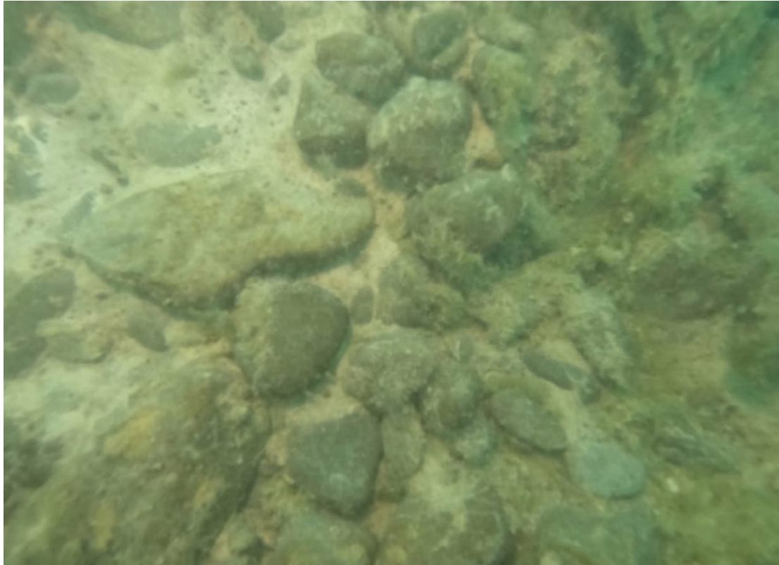
Figure 2-15. Example of exposed aggregate on rib surface (Rib 1).
