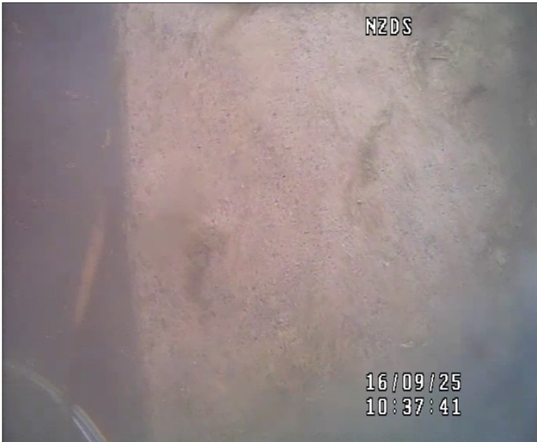
Figure 2-9. Typical condition of rib concrete (Rib 1).
