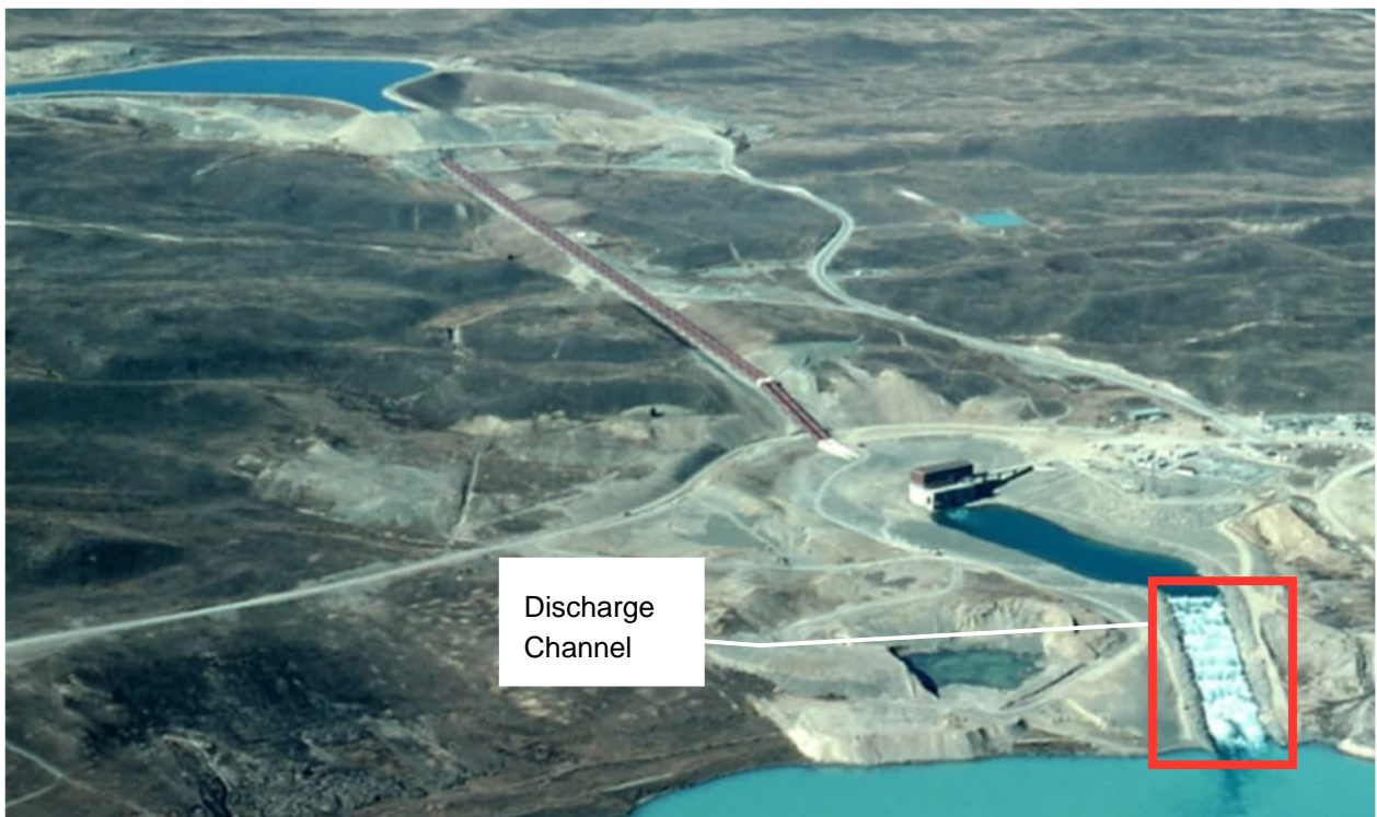
Figure 1-6. Photo of channel structure when Lake Pukaki is lowered.
