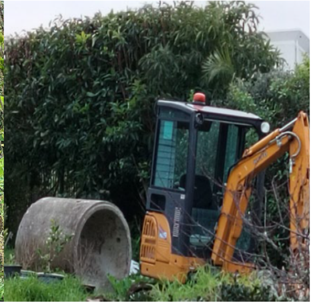
8. Pipe which replaced the drain
