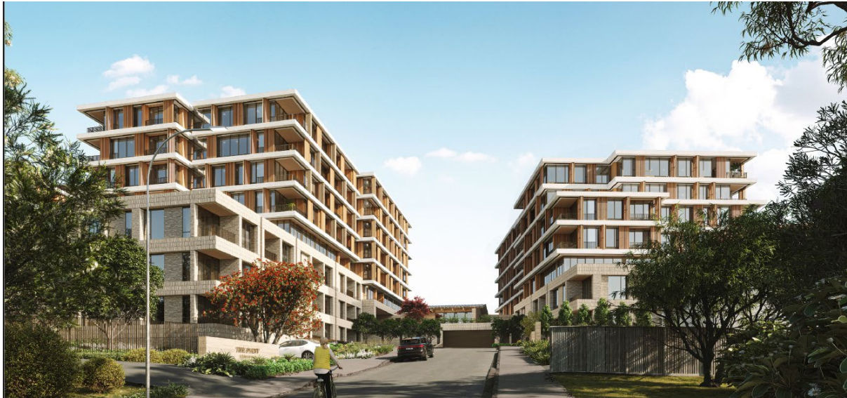
14. View of the proposed development from a favourable perspective at end of Rukutai St.
