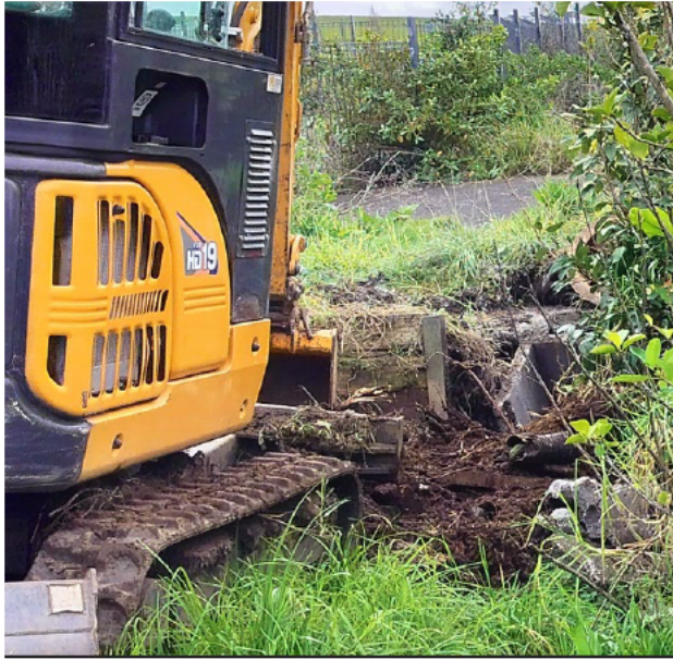
7. Drain being dismantled and removed
