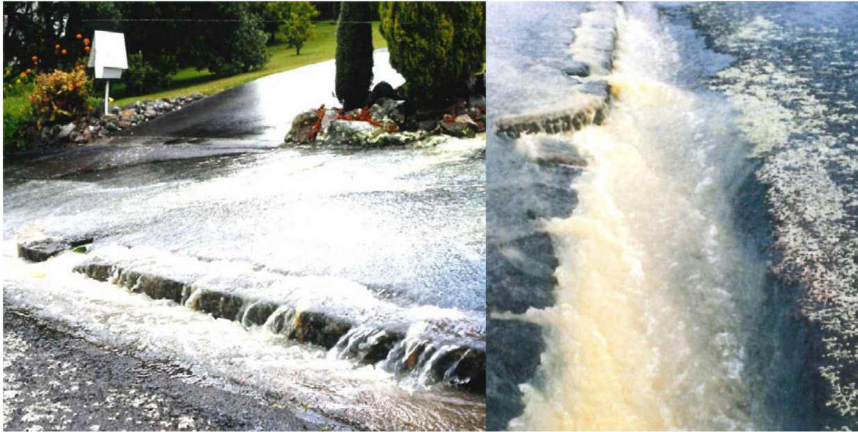
2. Water over footpath to kerbside from [REDACTED]
