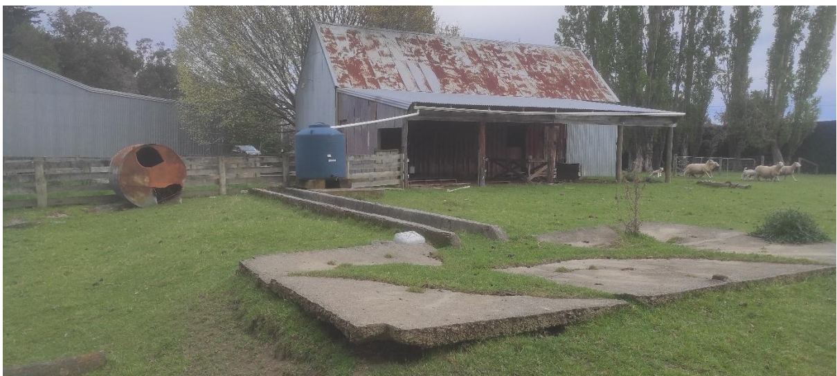
Figure 13: The sheep dip in the northern end of the site, leading from the yards to a concrete platform (17 October 2025).
