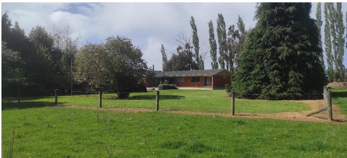
Figure 7: The existing dwelling at 270 Dukes Road North (16 October 2025).
