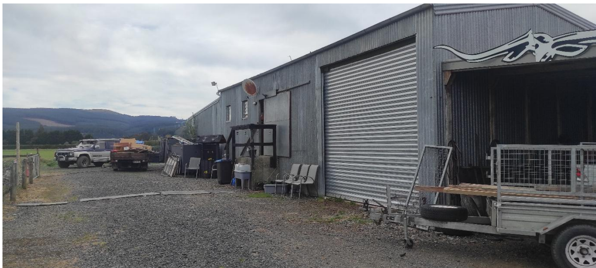
Figure 14: The woolshed in the centre of the site which has been converted into a workshop (17 October 2025).
