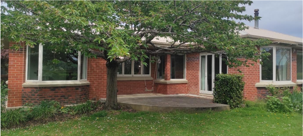
Figure 8: The existing dwelling at 274 Dukes Road North (17 October 2025).
