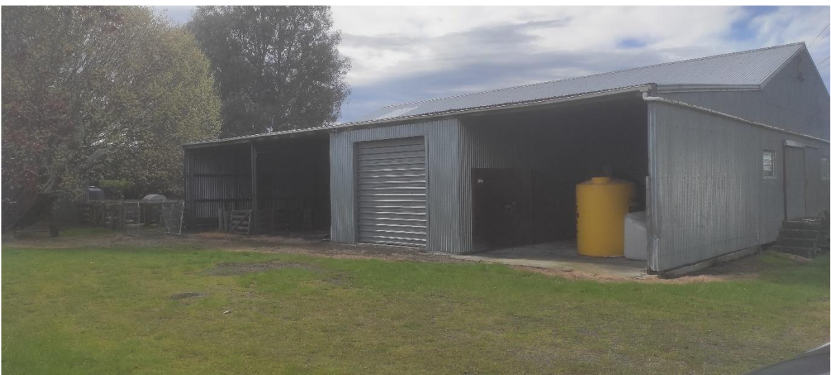
Figure 10: An example of one of the sheds present in the northern corner of the site (17 October 2025).
