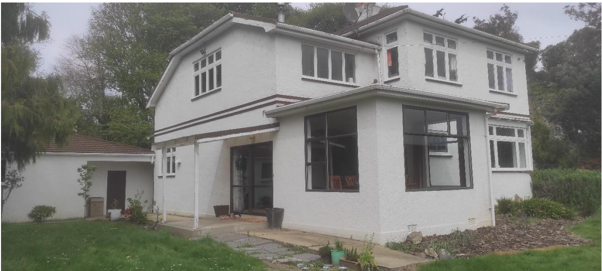
Figure 9: The existing dwelling at 292 Dukes Road North (17 October 2025).
