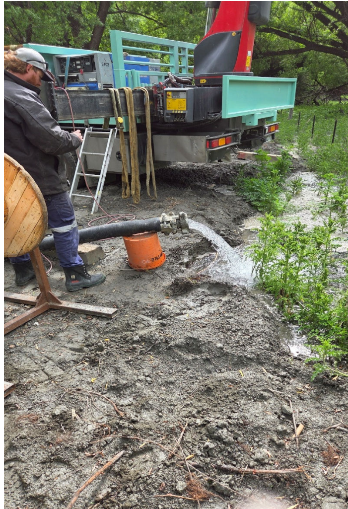
Photograph 3 Low turbidity water from Hole 5 near end of constant rate test.
