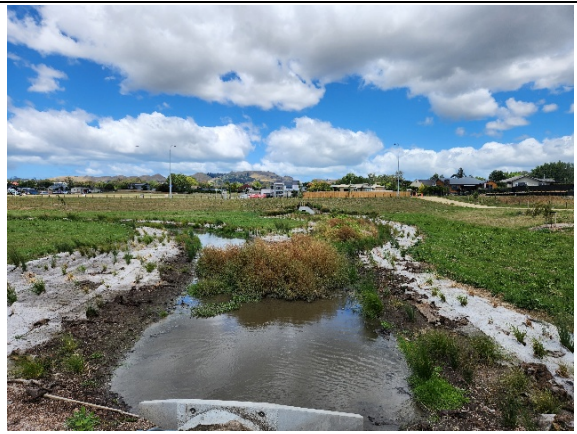
Photo 15. Stormwater management area for Iona subdivision, south of site. December 4, 2025.
