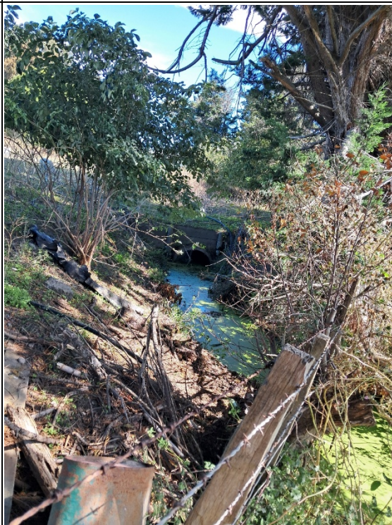
Photo 12. Farm drain on western boundary of McKenna Block. February 5, 2026.
