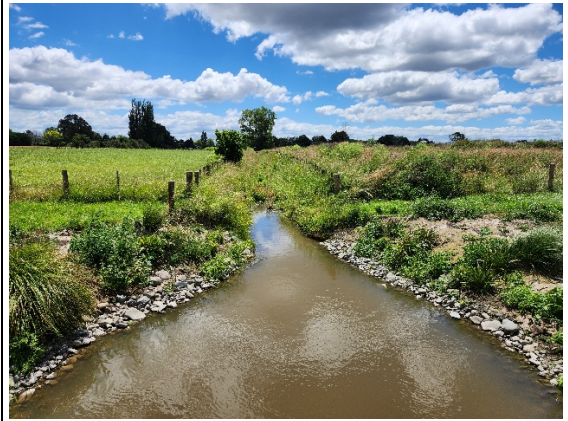
Photo 16. Outlet from stormwater management area for Iona subdivision, south of site. December 4, 2025.
