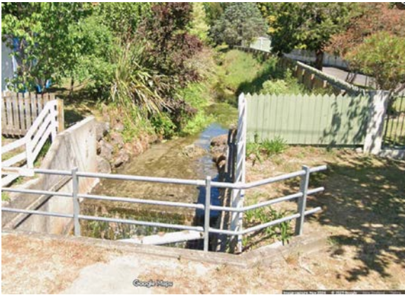
Photo 17. Herehere Stream At Reynolds Road (c. 500 m upstream of site). The vertical fall over 0.5m height is likely to impair fish passage. Google Streetview, 2024.
