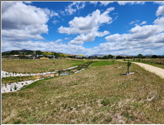
Photo 14. Stormwater management area for Iona subdivision, south of site. December 4, 2025.
