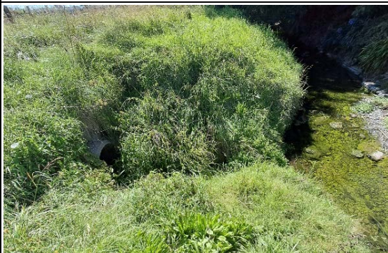
Photo 13. Farm drain outlet into Herehere stream. February 5, 2026.
