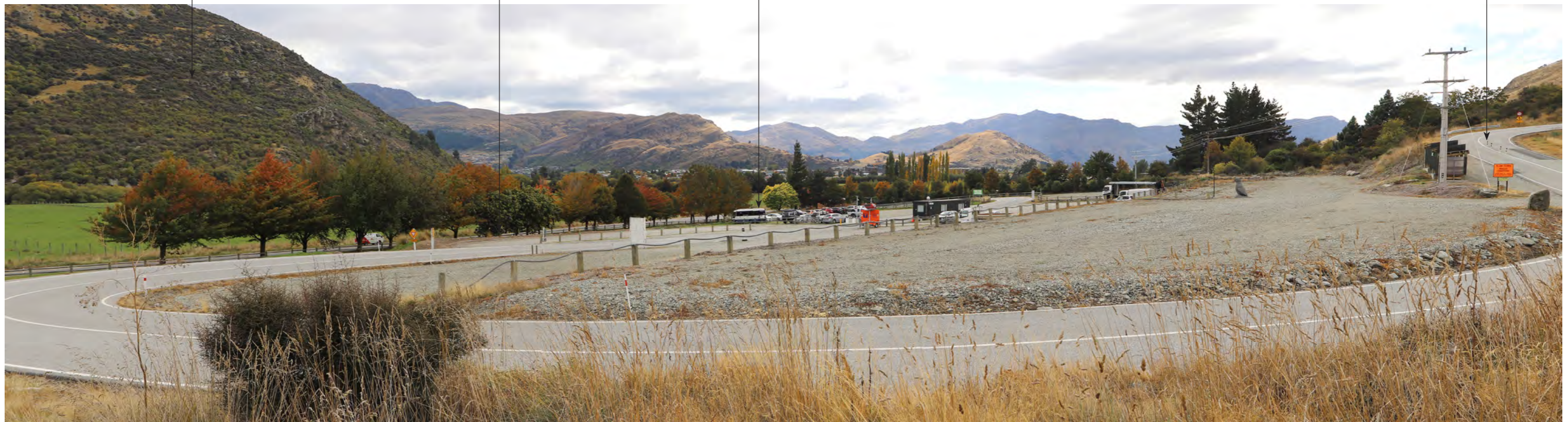
Site Photograph 4: Photograph of existing carpark A, looking in a northerly direction
