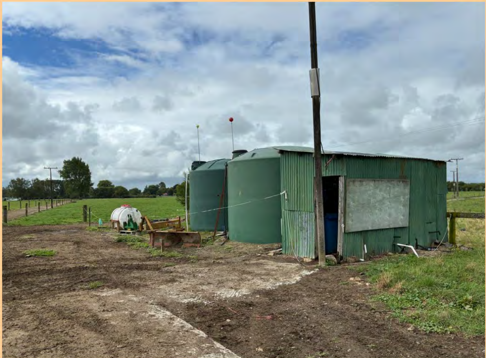
20 Montgomeri e Farm: Pump shed
