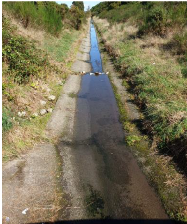
Figure 29: Main drain as seen from atop headwall outlet
