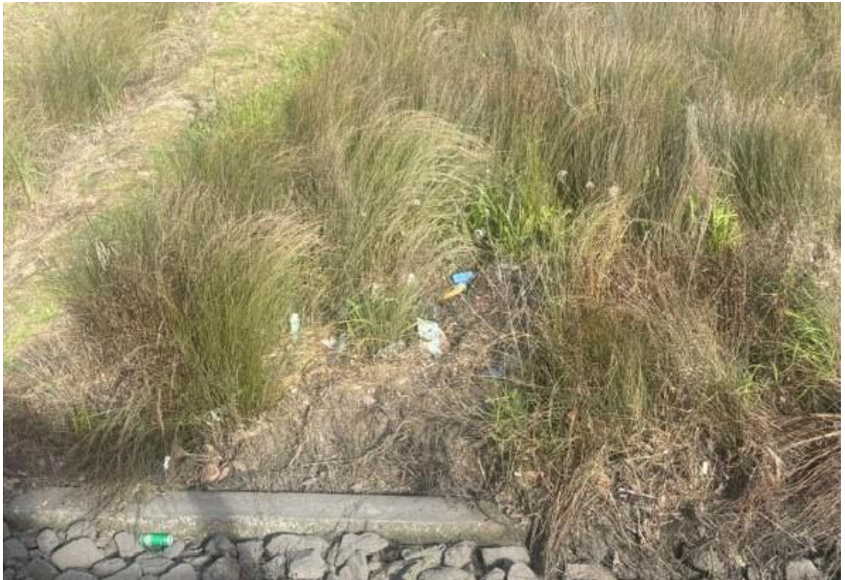
Figure 3. Sediment and Litter Accumulation in Wetland Swale
