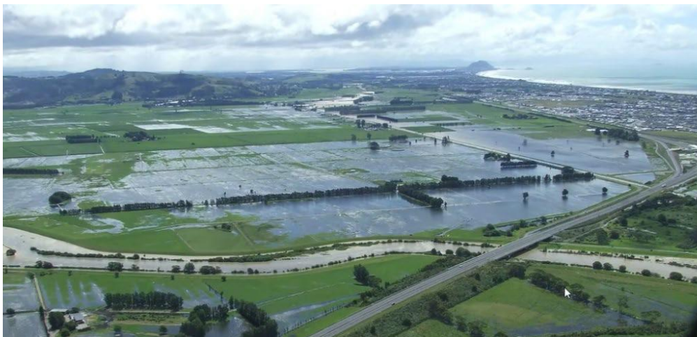
Figure 1: Flooding on 23 January 2026 (approximately 220 to 250 mm of rainfall on 21-22 January 2026)
