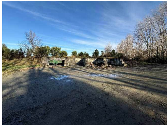
Photo 5: Concrete block storage bunkers possibly used for fertiliser
