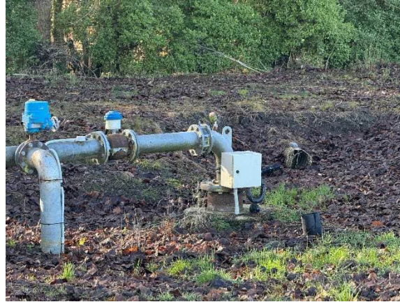
Photo 8: Existing well bore in facility maintenance compound
