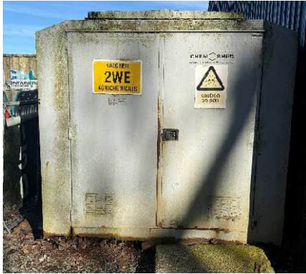
Photo 7: Agrichemical Storage in compound
