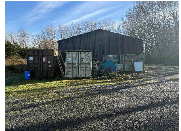
Photo 6: Facility Management Compound and HSNO shed
