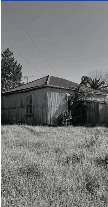
Existing rural structures on the Surfpark Site
