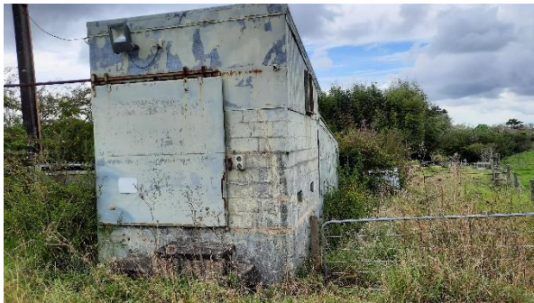
Photograph 3: Livestock farm structure
