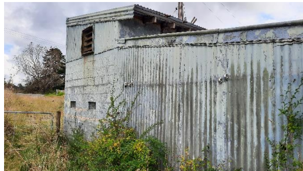
Photograph 4: Southern side of the livestock farm structure
