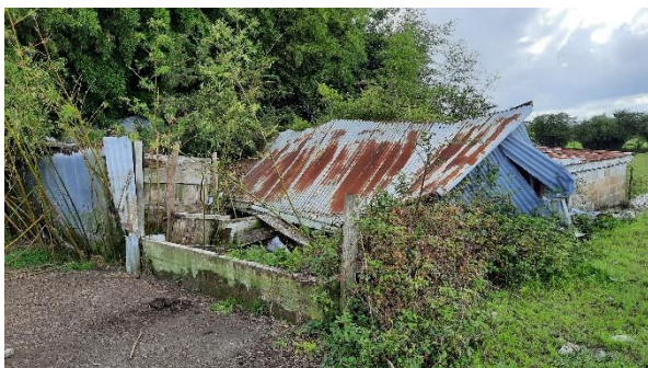
Photograph 7: Collapsed farm structure
