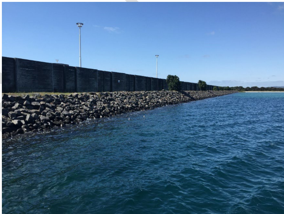
Photo 1: Riprap revetment along Northport western boundary
