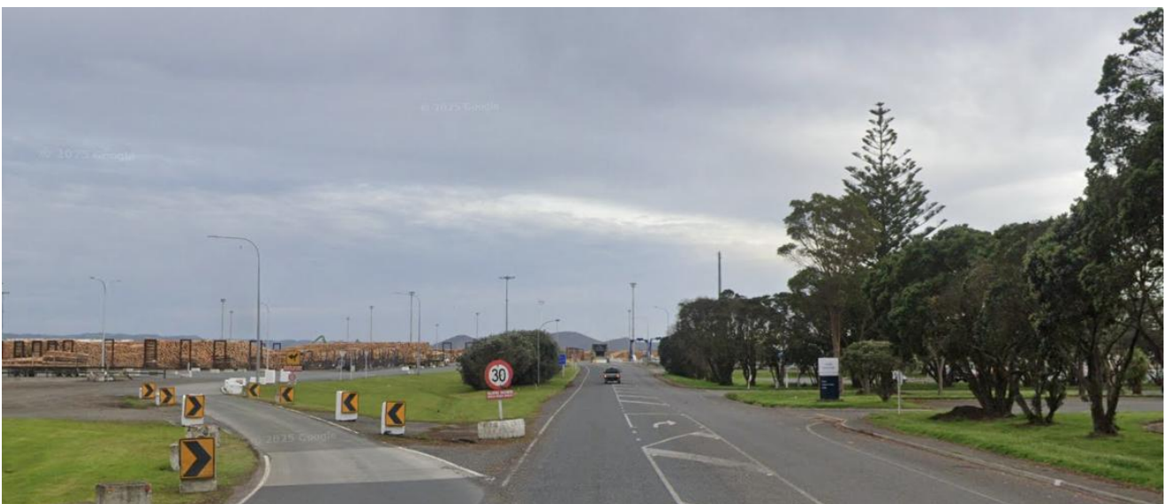
Figure 6: Port Marsden Highway looking north towards the existing port facility (source: Google Street View October 2025)
