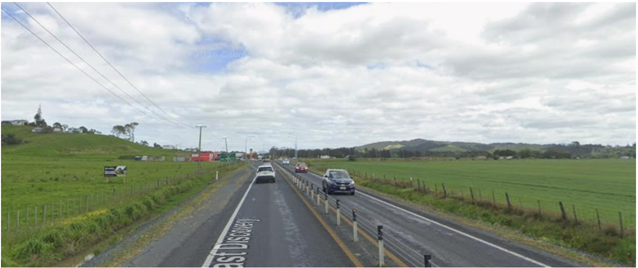
Figure 5: SH1 looking towards to SH1/Port Marsden Highway intersection (source: Google Street View October 2025)
