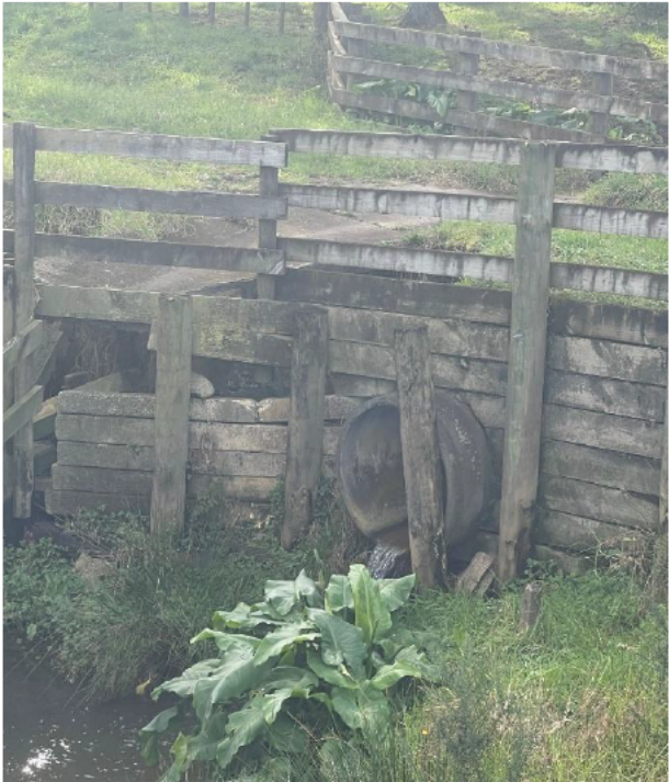
Figure 2 Western Culvert (perched), looking north-east across farm track
