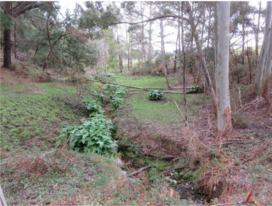
Figure 4 Eastern Culvert outlet looking west downstream
