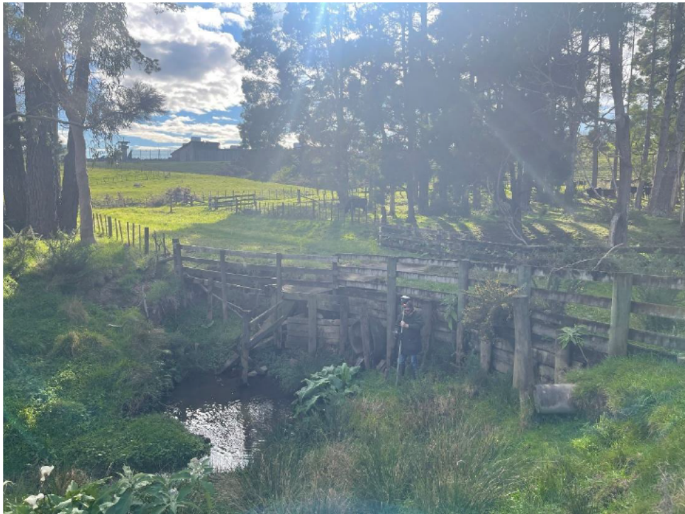
Figure 1 Western Culvert, taken from 43 Merewhira Road, looking north-east
