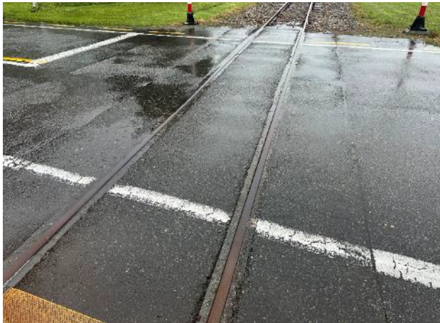
Figure 3-11: Track panel in good condition
