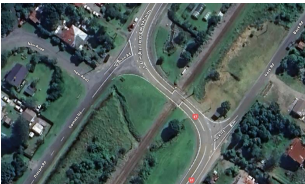
Figure 3-2: SH67 Granity Ngakawau level crossing aerial (Source: Google Maps)
