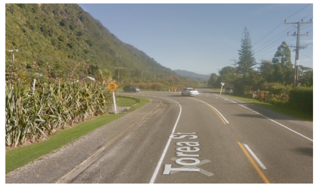
Figure 3-10: Vegetation masking the approach of southbound trains (Google Street View)
