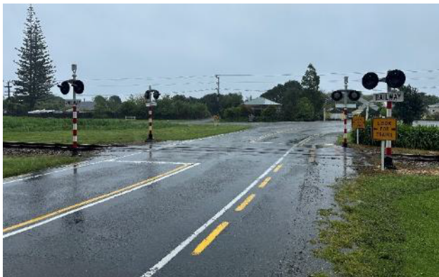
Figure 3-3: Southern approach to the level crossing from Torea Street
