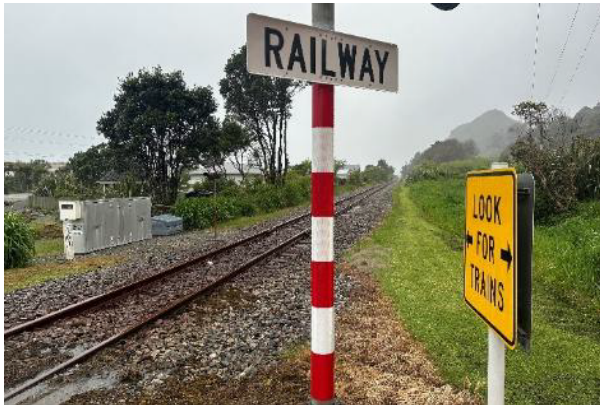
Figure 3-5: UP track sightline on southern approach
