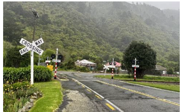
Figure 3-4: Northern approach to the level crossing from Torea Street
