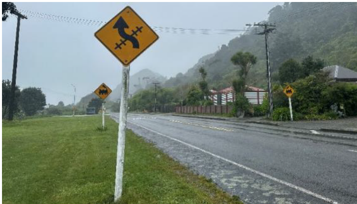
Figure 3-18: Level crossing alignment sign from southern approach
