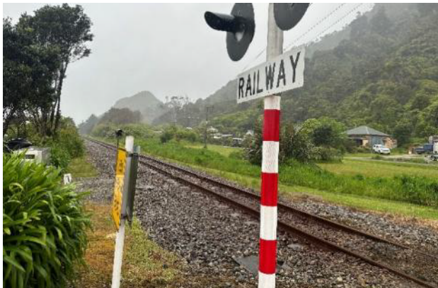
Figure 3-7: UP track sightline on northern approach
