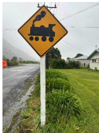
Figure 3-17: WX1R sign on northern approach
