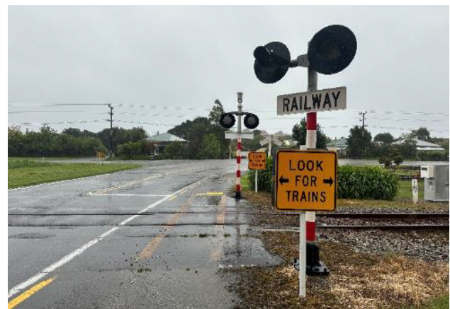
Figure 3-26: Pedestrian crossing southern approach
