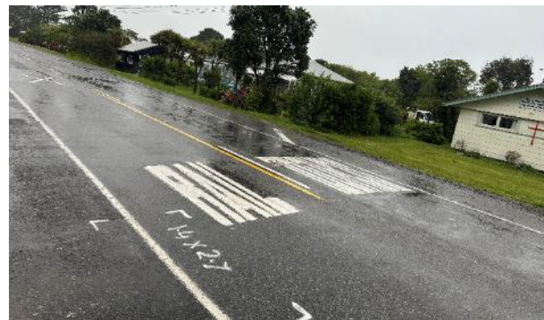
Figure 3-20: Rail X markings from northern approach
