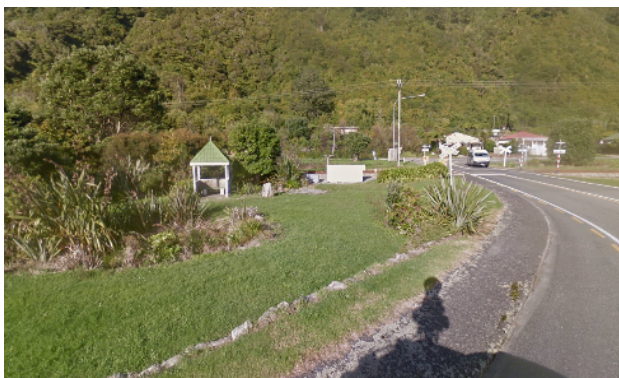
Figure 3-9: Poor visibility of crossing controls from the north (Google Street View)
